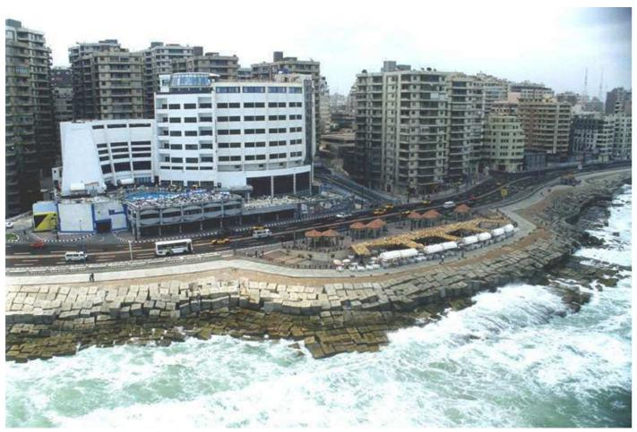
Concealing the waterfront with the cordon of concrete blocks induces the rise of wave altitudes to hit the concrete blockage on the waterfront.
