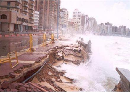
Damage at Mandara beach during the storm in 2003. The sand beach was vanished with wave scouring underneath the road seawall.
