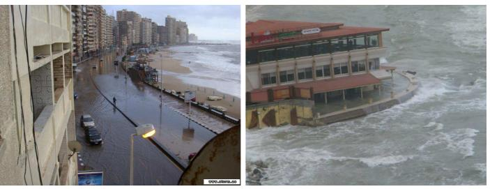
Because of the low level of the road, it was immersed by the sea during the storm, but with no damage due to the submerged breakwater. Refer to Map 4: Part 2.
