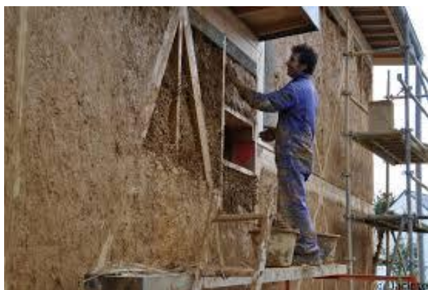
15.3.4a Posa in opera
