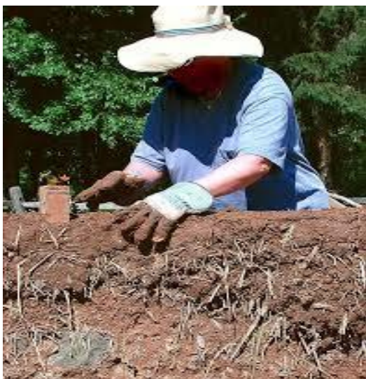
15.3.3a Posa in opera
