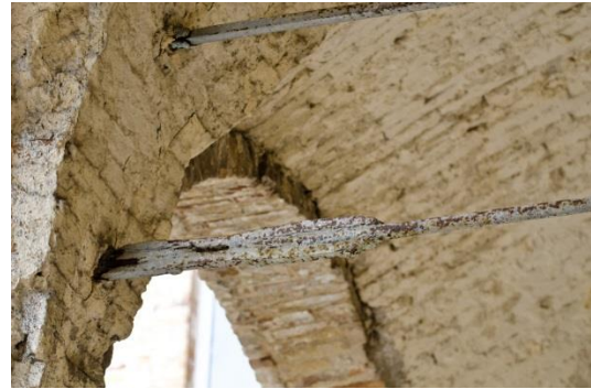
Fig. 1-3: tie-rods in Recanati (MC) - Italy
