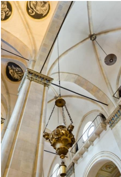
Fig. 1-4: tie-rod with added mass in Loreto's Basilica (AN) - Italy
