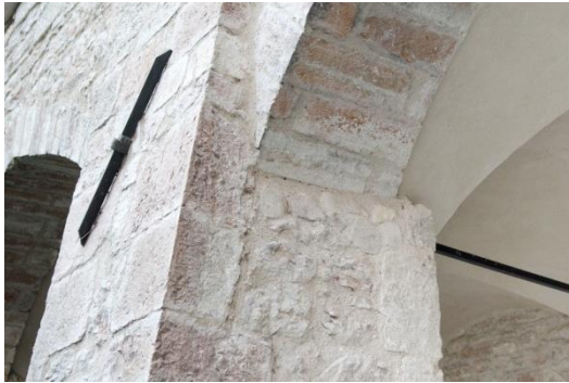
Fig. 1-2: tie-rods in Visso (MC) - Italy
