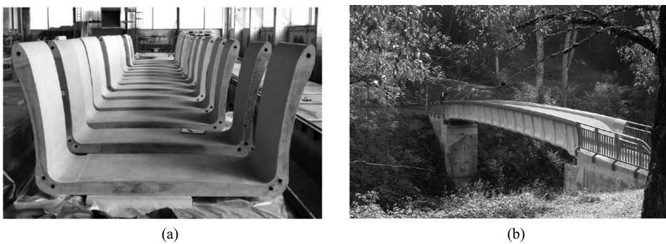
Figure 3.14: U-shaped TRC pre-fabricated elements (a) and assembled bridge placed in Kempten (b) [Curbach and Sheerer (2011)].
