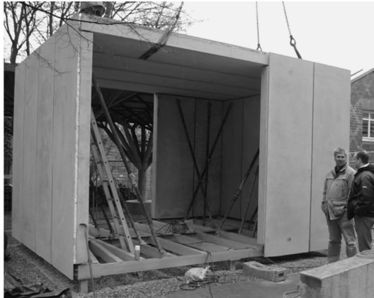
Figure 3.12: Assembly of modular prototype TRC sandwich building [Hegger and Horstmann (2009)].
