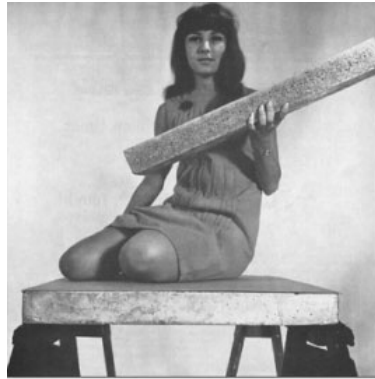
Figure 1.29: Bjorksten demonstration of both lightness and stiffness of Al foams [8].
