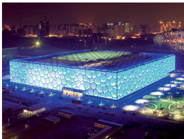
Figure 1.3: The Beijing National Aquatics Center, also known as the Water Cube, was built for the swimming competitions of the 2008 Summer Olympics. The outer wall is based on the Weaire-Phelan structure, a structure devised from the natural pattern of bubbles in soap lather [63].
