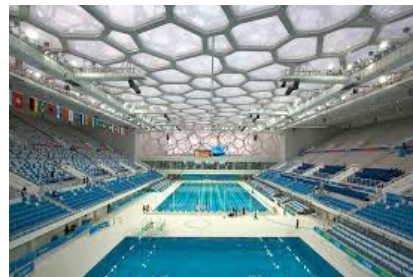
Figure 1.3: The Beijing National Aquatics Center, also known as the Water Cube, was built for the swimming competitions of the 2008 Summer Olympics. The outer wall is based on the Weaire-Phelan structure, a structure devised from the natural pattern of bubbles in soap lather [63].
