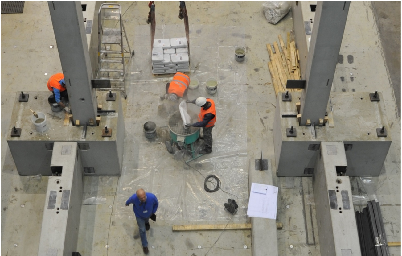
Figure 5.31 – Pocket column-to-foundation connections
