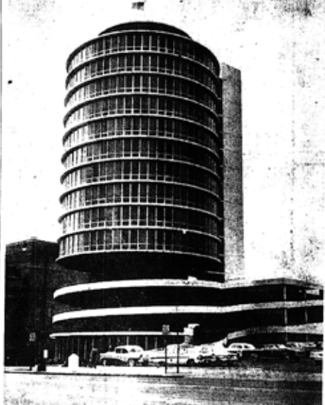
The Christopher Lane, 25-story office tower, has parking space on second, third and fourth levels.
