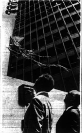
AWAY IT GOES: The last bucket of concrete heads towards the top of Place Victoria, as Mayor Jean Drapeau and George Hees, chairman of the Montreal and Canadian Stock Exchange look on. A few moments before they had pressed a button, starting an electronic relay that would hoist the bucket to the top and pour the last of the concrete.
