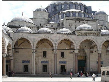
Fig 2.221: 'Süleymaniye Mosque arches and columns', 1856, Istanbul (Wikipedia.org, 2012).
