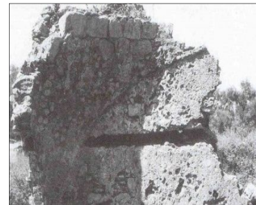
Fig 2.75: Tomb in Perçin, use of timber tie beam outside leaves of the masonry wall (Kolay, 1999). Fig 2.76: Tomb in Perçin, use of timber tie beam inside leaf of the masonry wall (Kolay, 1999). Fig 2.77: Tomb in Perçin, timber tie beam hole outside leaves of the masonry wall (Kolay, 1999).
