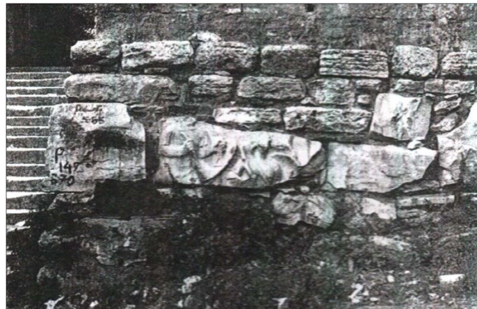
Fig 2.211: Picking material use from ancient structures, detail (Beyazit Hamami, 1506-1507) (Akinci, 1998).
