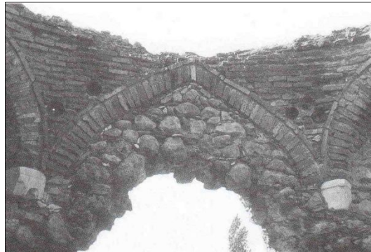
Fig 2.82: Tomb in Perçin, wall pattern and pendentive ( Kolay, 1999 ).
