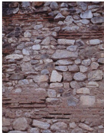
Fig 5.6: Traces of offset in historical walls surrounding znik (south wall) (Adatepe, Erel 2006)
