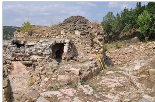
Fig 7.4: Emirler bath south-west view (Endowment office Bursa, 2012)
