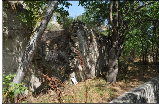
Fig 7.17: Süleymanpa a bath south wall view 2
