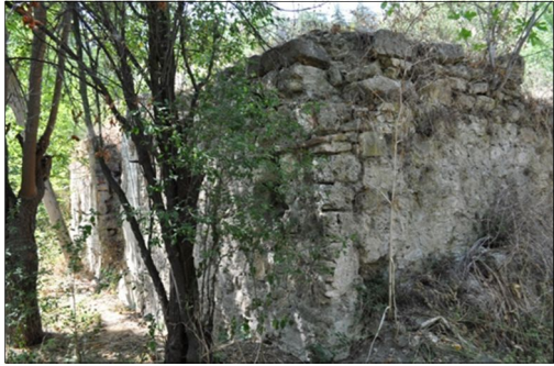
Fig 7.16: Süleymanpa a bath south wall view 1
