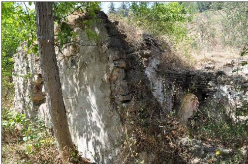
Fig 7.18: Süleymanpa a bath south wall view 3
