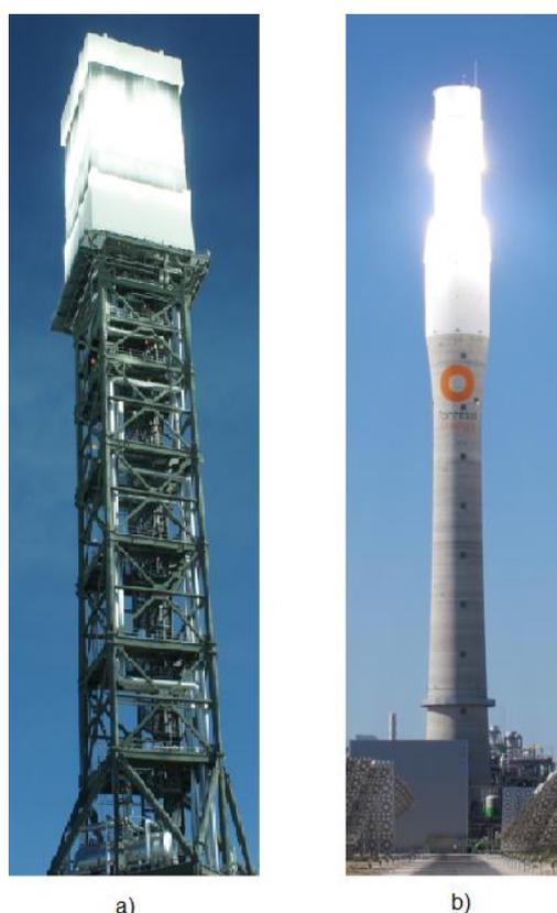
Figure 1. 7. Steel lattice vs Concrete Tower. a) Ivanpah, b) Gemasolar.
