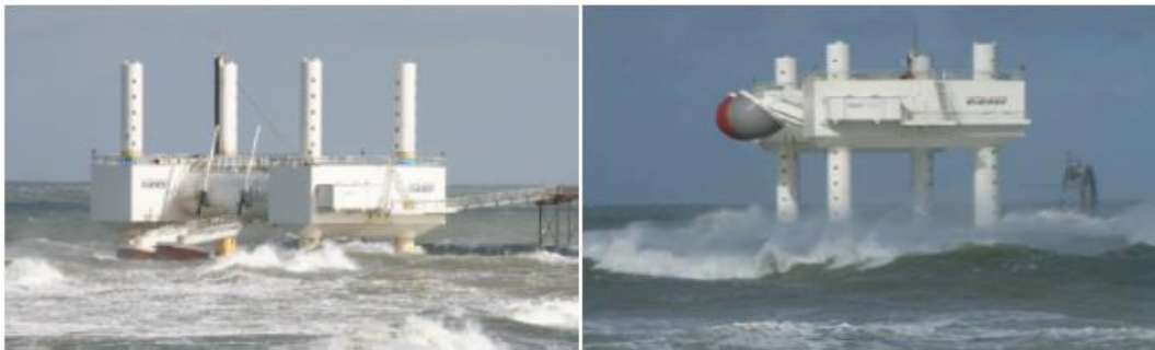
Figure 2-1 Wave Star in Production and Storm Protection
