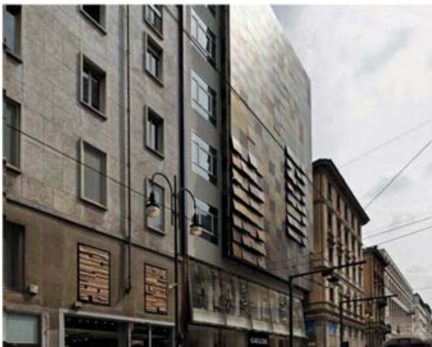
Fig.068 Breatbuilding, via Torino - Dante Benini & Partners
