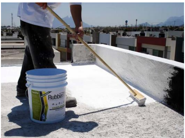
Figure 5- 5 White water proof layer made of recycled tires
