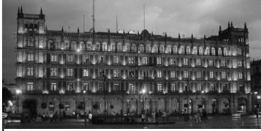
Figure 2- 44 Mexico City's hall
