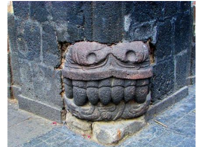
Figure 2- 18 Reuse of prehispanic stone in colonial building
