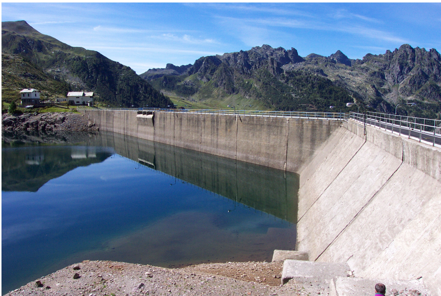
Figure 3.11: Pescegallo reservoir, source: ARPA Lombardia
