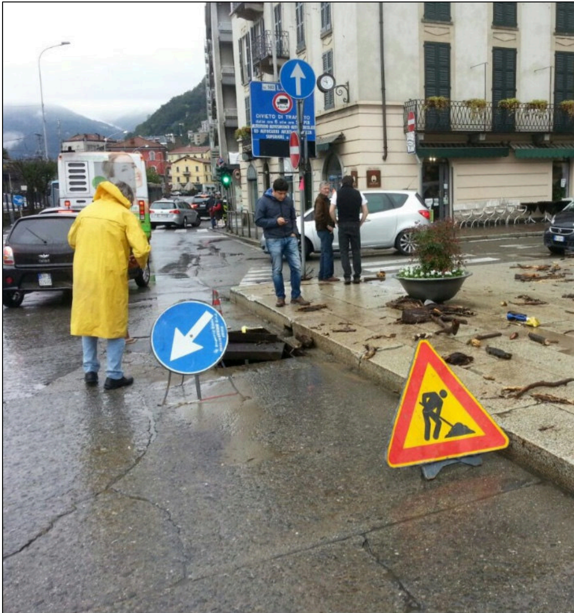
Figure 56: 11/ 10/ 2014, Valduce uplift manhole after intense rainfalls (QuiComo).
