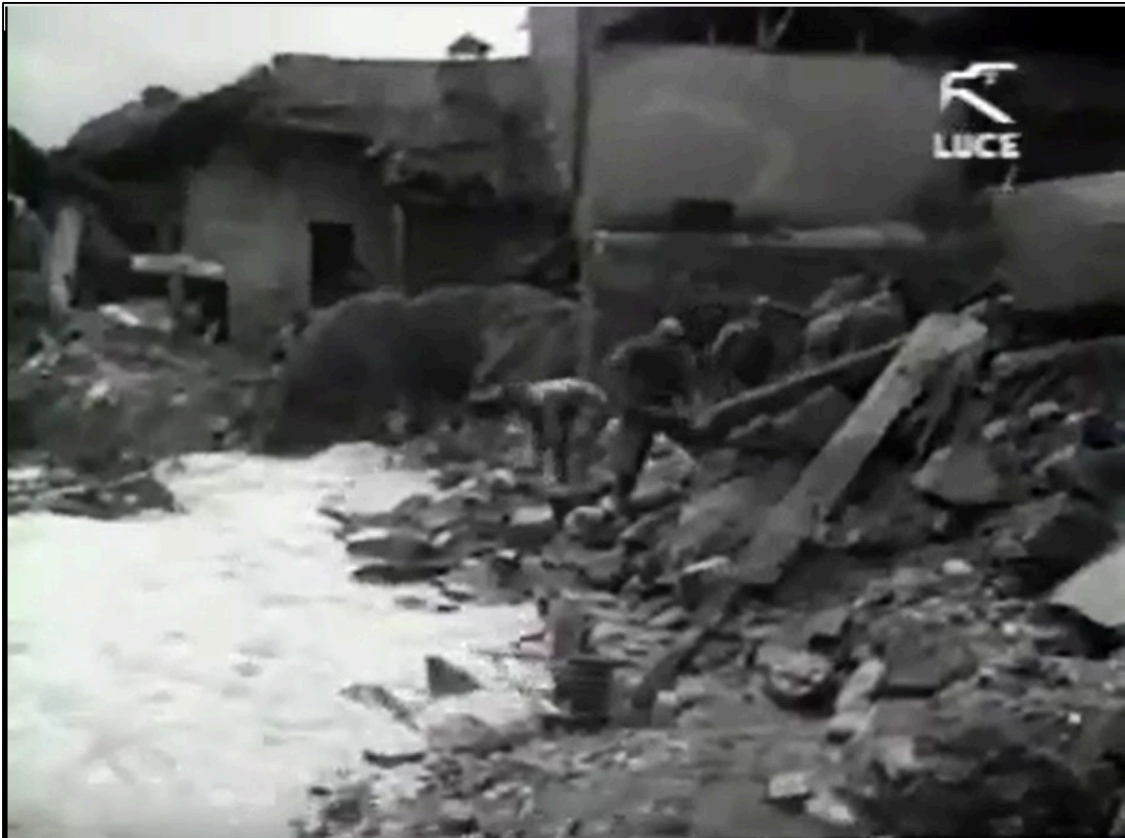
Figure 57: Landslide on Cosia Torrent, 1951 (Archivio Storico Istituto LUCE).
