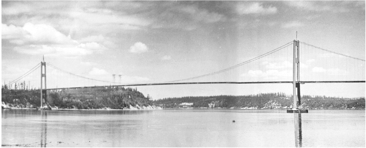
Figure I.27_Tacoma Narrow Bridge.
