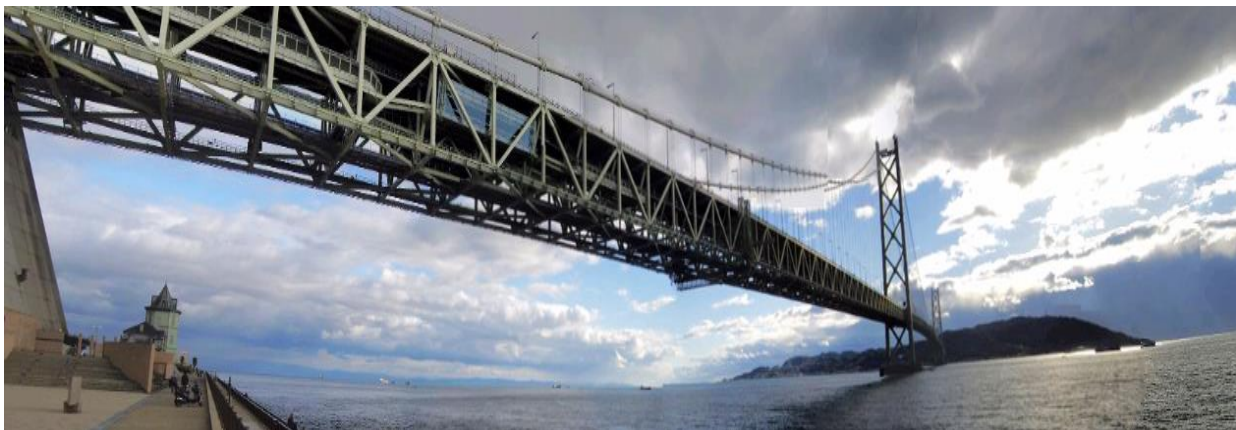
Figure I.32_Akashi Kaikyo Bridge.
