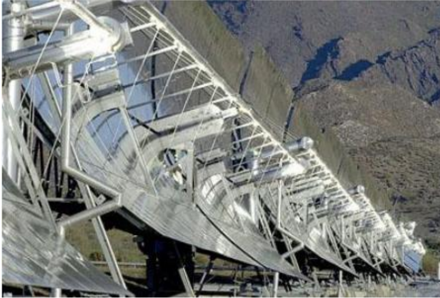
Figure 1-4 The collector field of the German/Spanish Direct Solar Steam (DISS) project (Badr, 2013).
