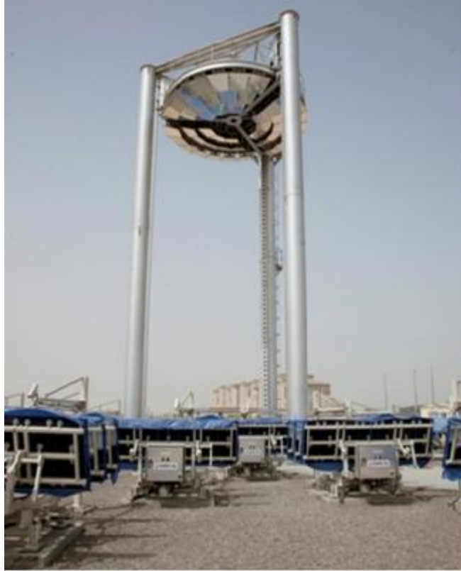
Figure 1-6 The Beam-down solar concentrator in Masdar City, Abu Dhabi, UAE (Badr, 2013).
