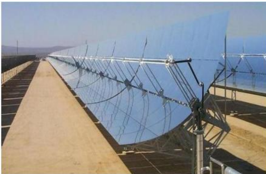
Figure 1-3 Installation of parabolic trough collector at the SEGS V, California (Badr, 2013).
