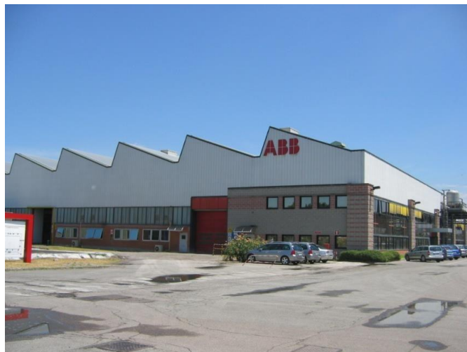
Figure 1: ABB factory in Vittuone (MI).
