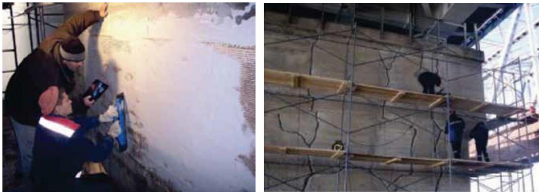
Figure 1. 17 - Strengthening of reinforced concrete bridge pier
