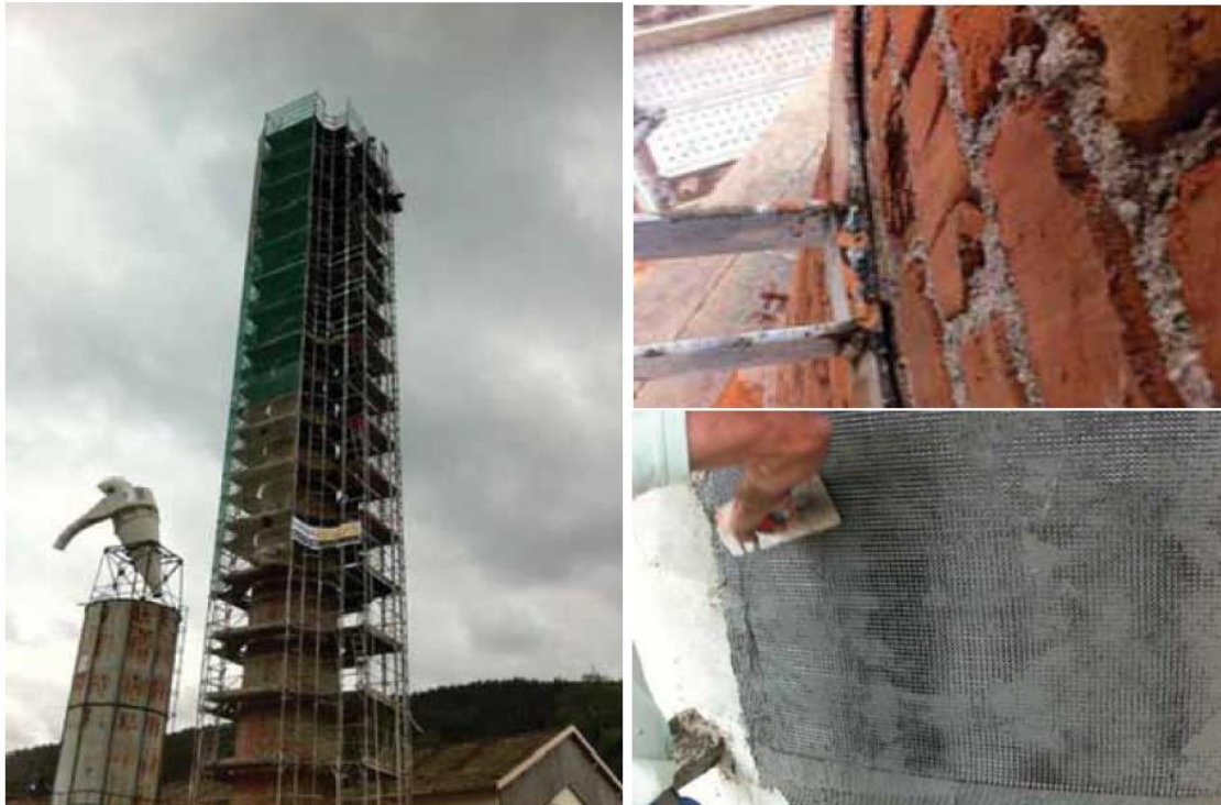
Figure 1. 16 - Strengthening of unreinforced masonry chimney
