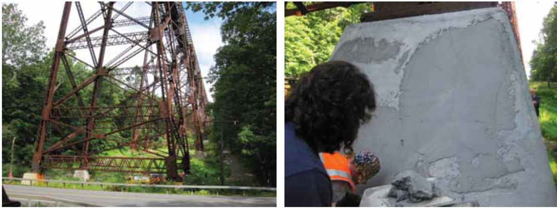
Figure 1. 14- Trestle bridge base
