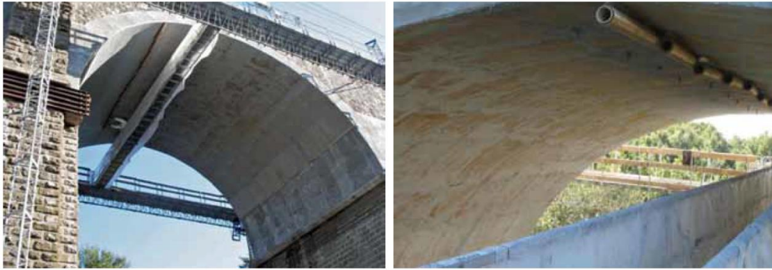
Figure 1.13-Unreinforced concrete vault strengthening
