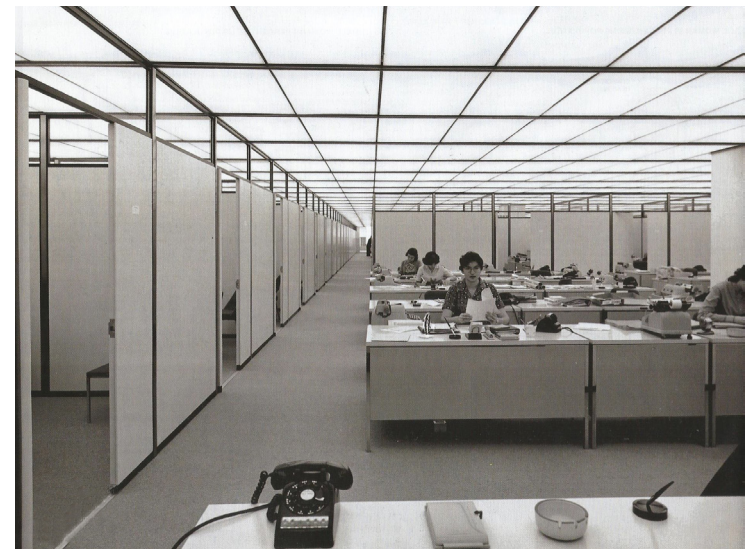
Union Carbide Building. Skidmore. New York. 1960
