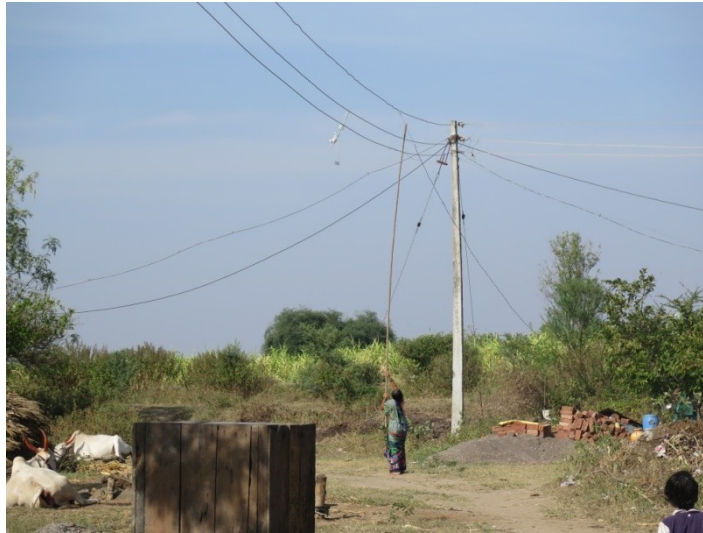
Fig. 3.1: Example of illegal connection to the electric grid
