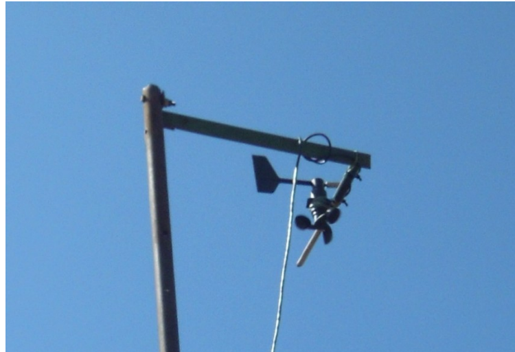
Fig. 4.2: Power Predictor installed in Katgaon
