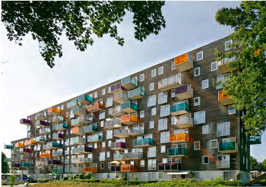
Figure 8-37 The street view of Wozoco (source from http://www.mvrdiv.nl )
