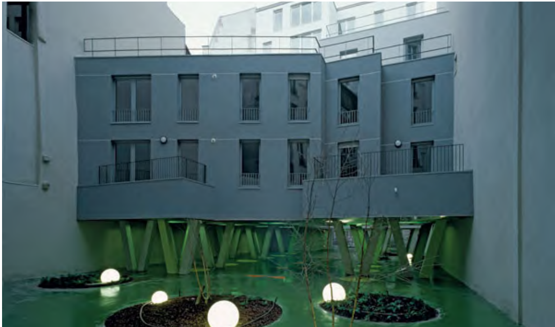
Figure 8-11 The view from the courtyard of Rivp Louis Blanc (source from archdaily)
