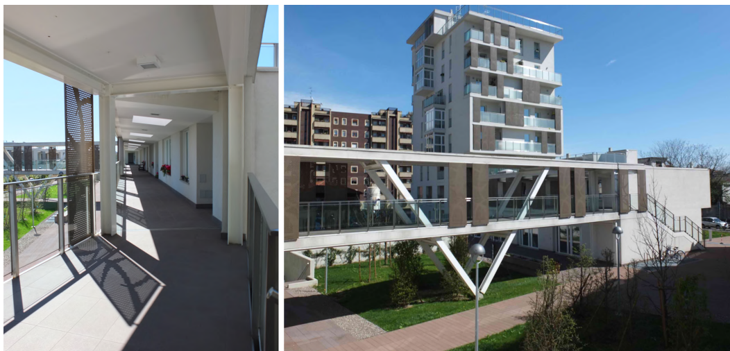
Figure 8-59 Connecting element of social housing in via Cenni (photo by authors)
