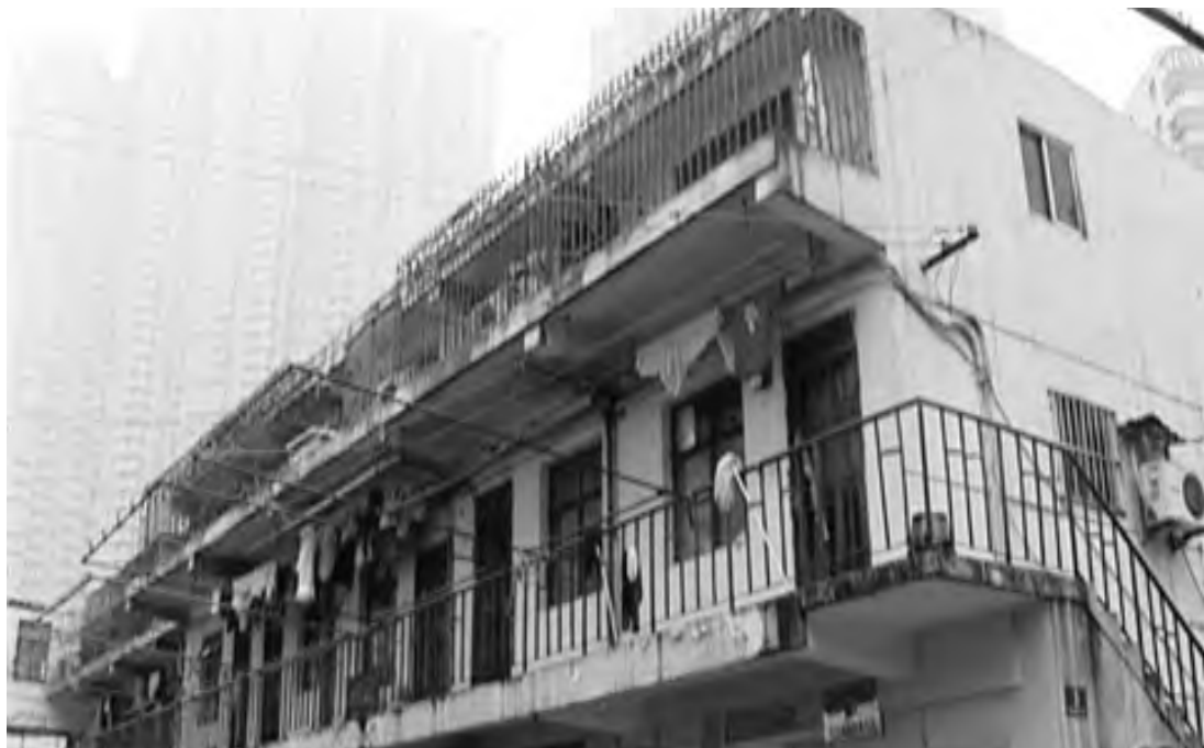
Figure 4-10 Exterior scene of "Yuanyang residence" (source from internet)
