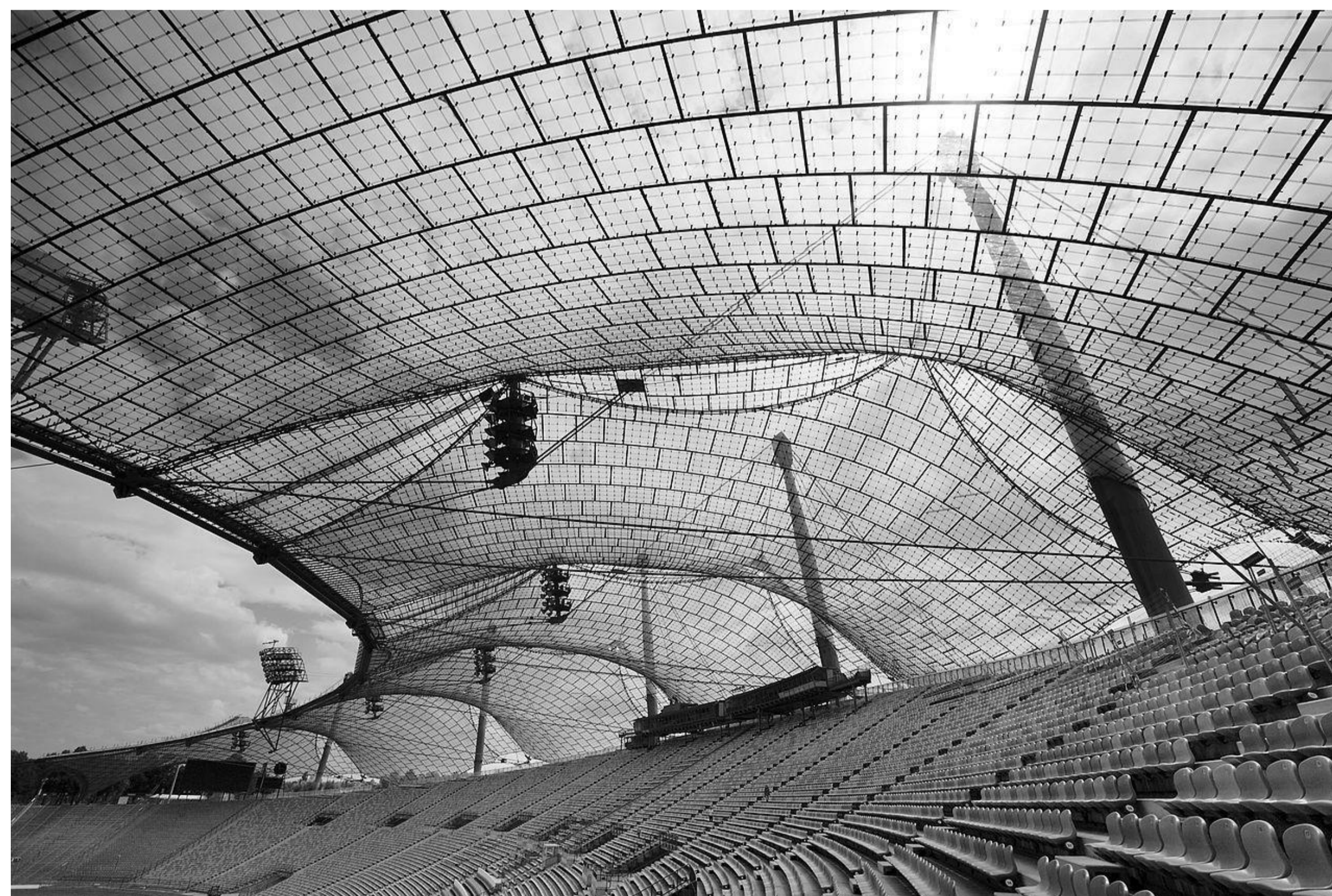
Figure 4) Interior grandstand roof structure of the Olympic Estate in Munich 1972
