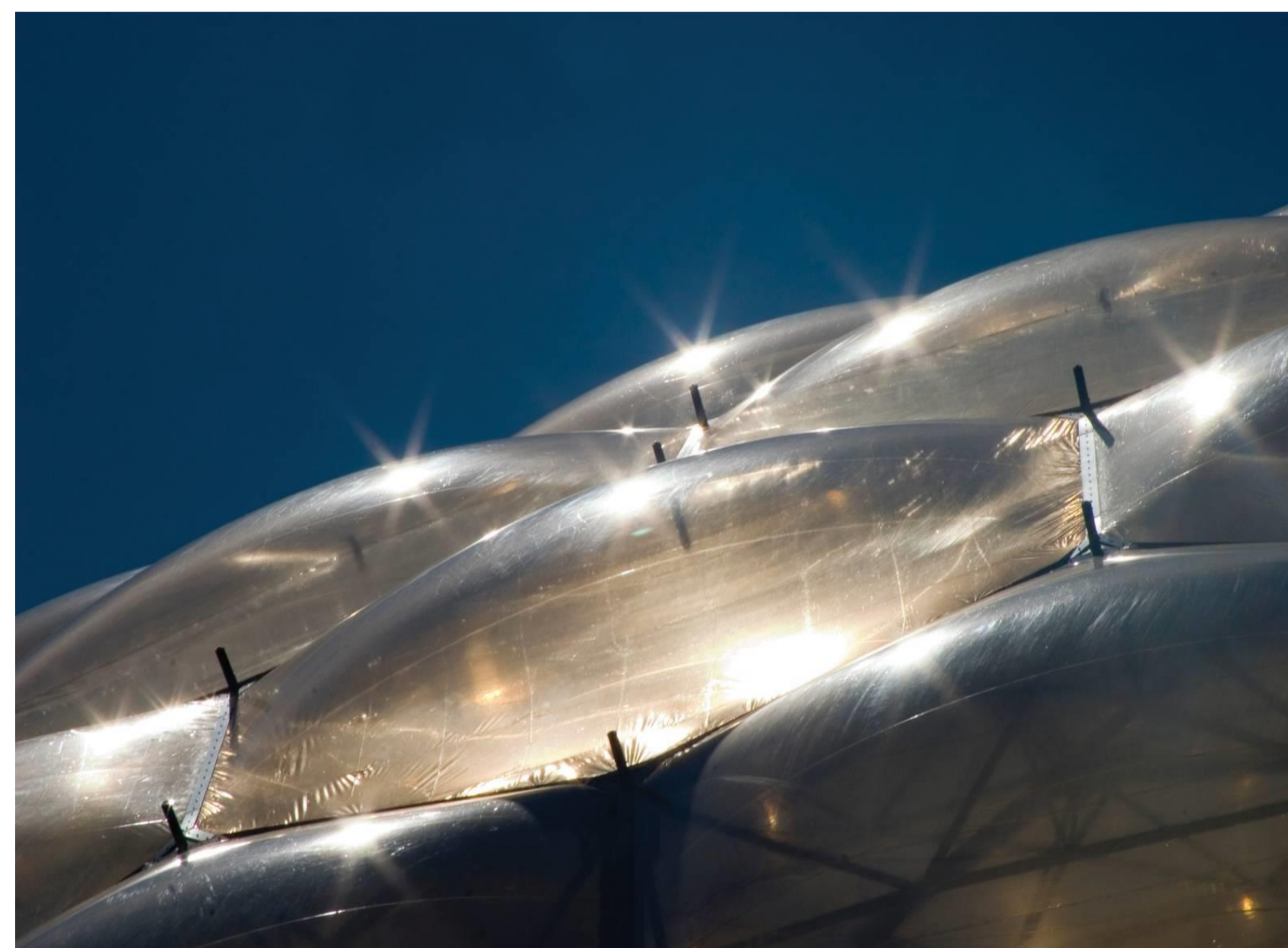
Figure 209) ETFE cushions
