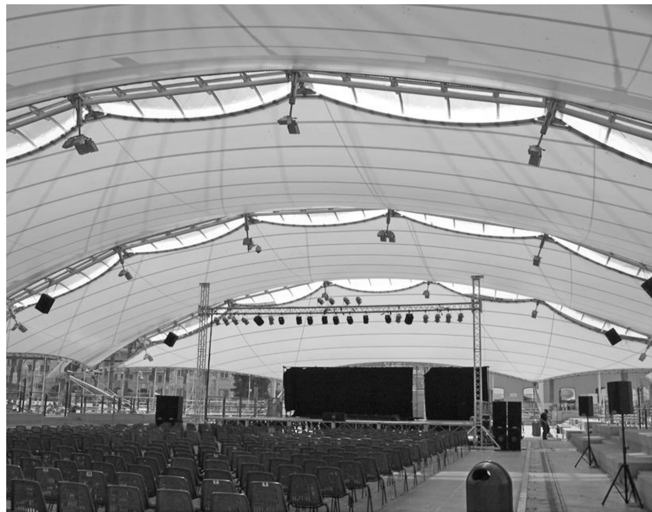
Figure 77) Light Patches due to direct light through the transparent areas, cast onto the inside of the membrane of the Bigo Tent.
