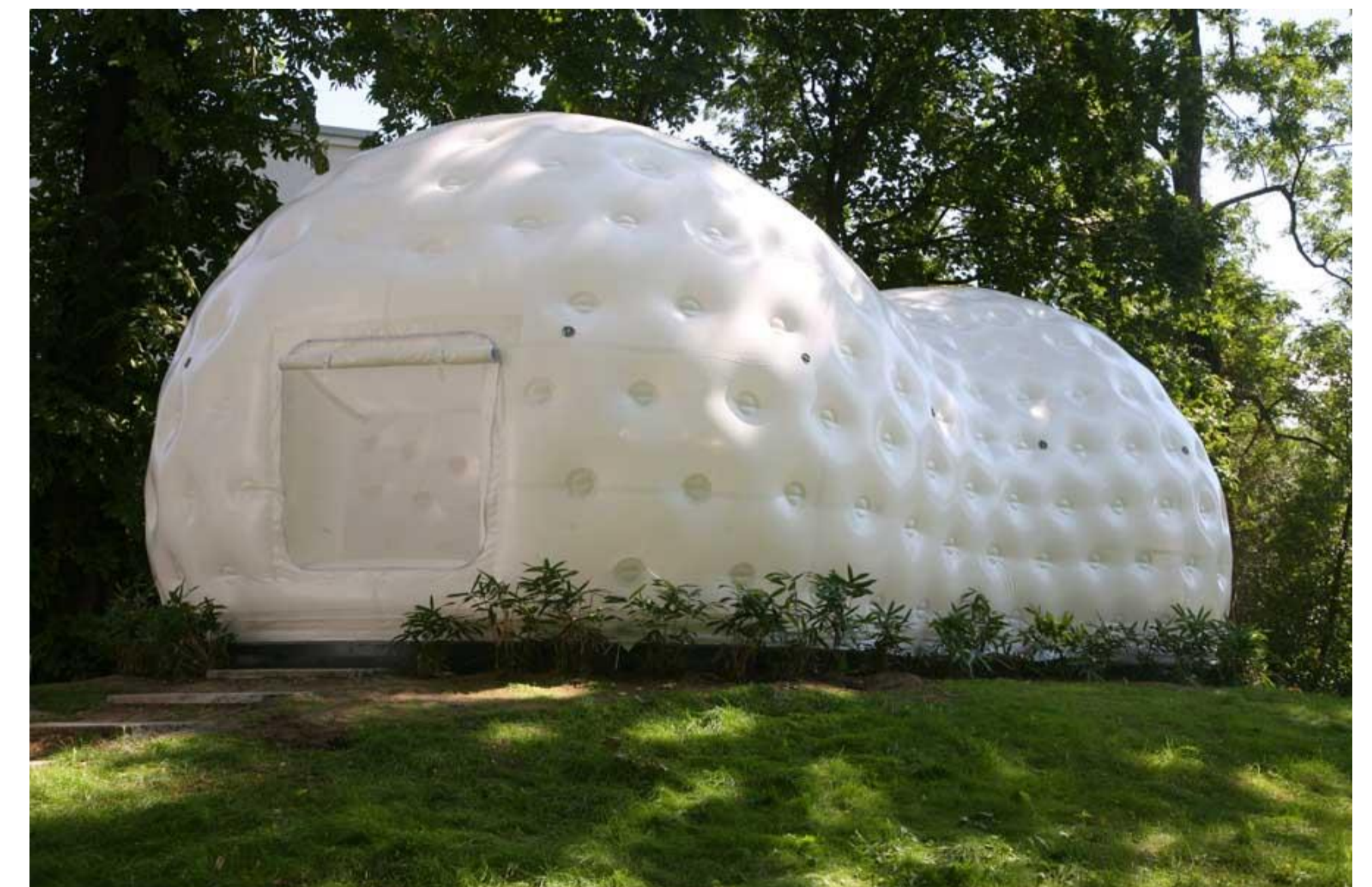
Figure 72) Inflatable Teahouse: Traditionally the Japanese tea house would be made with natural materials such as wood, bamboo, and rice paper, but Kuma has used a High-Tec fabric ,Gore Tenara, as a replacement. The fabric is sufficiently flexible to allow the structure to be deflated and inflated many times, enabling it to be moved as required. Garden Museum , Frankfurt 2007
