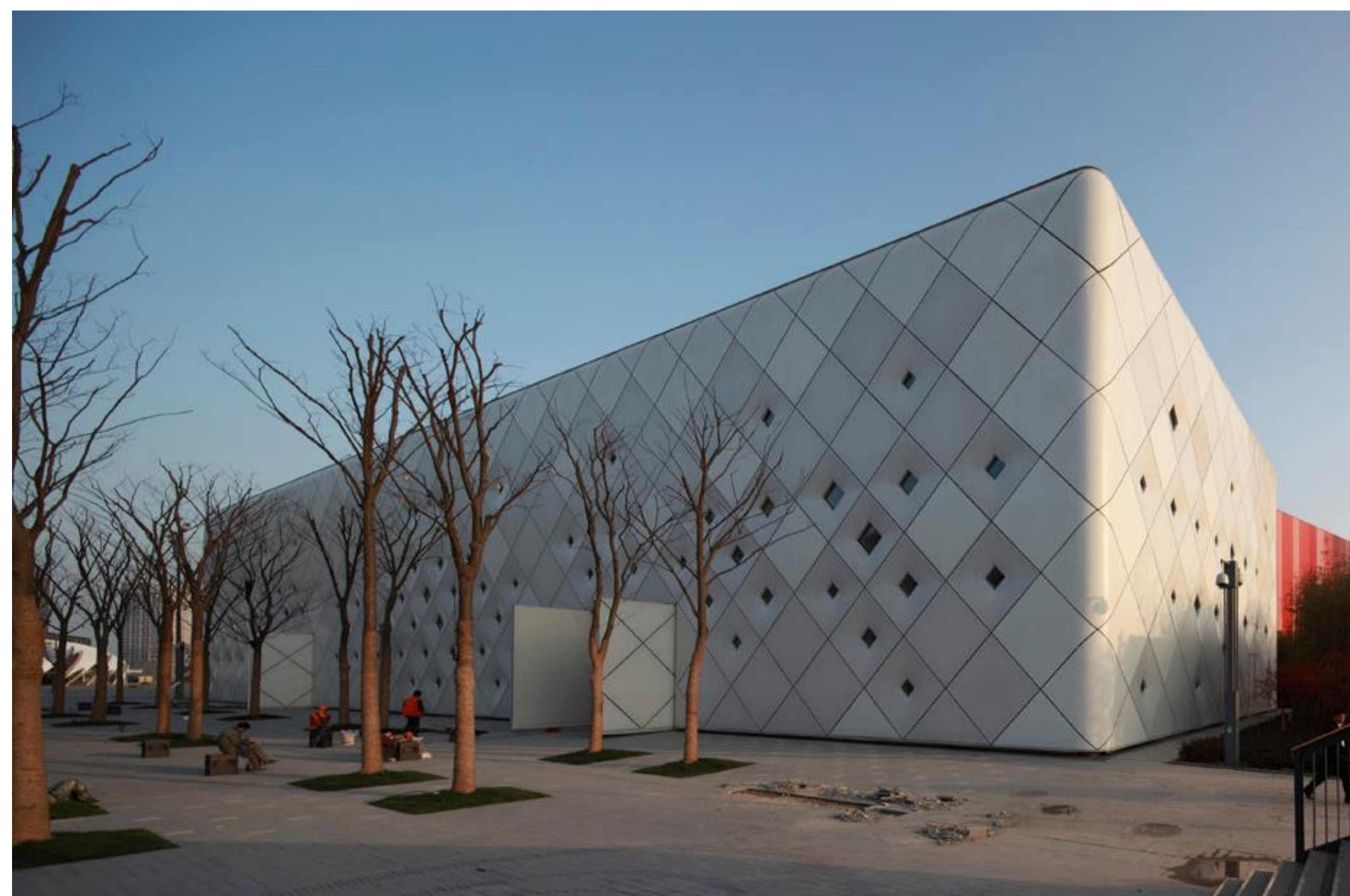
Figure 106) Italian Pavilion, Shanghai, Expo 2010
