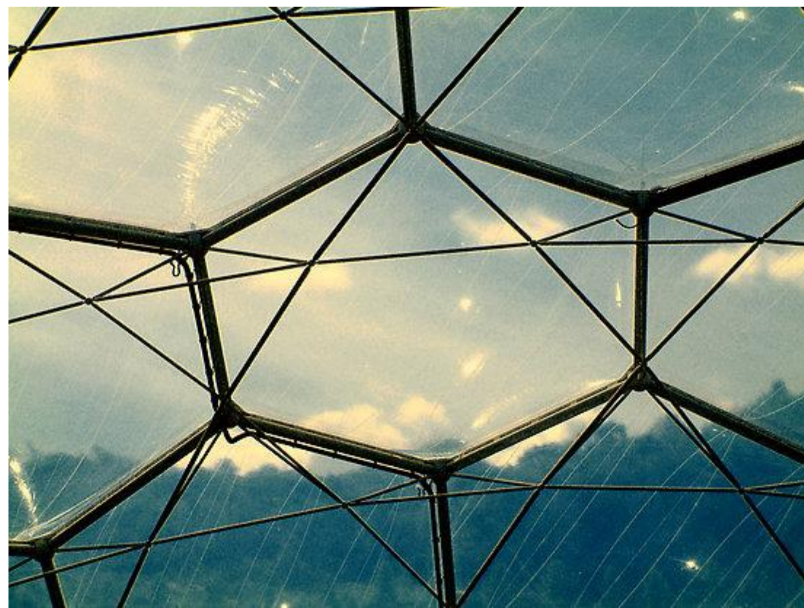
Figure 202) Inside looking out
