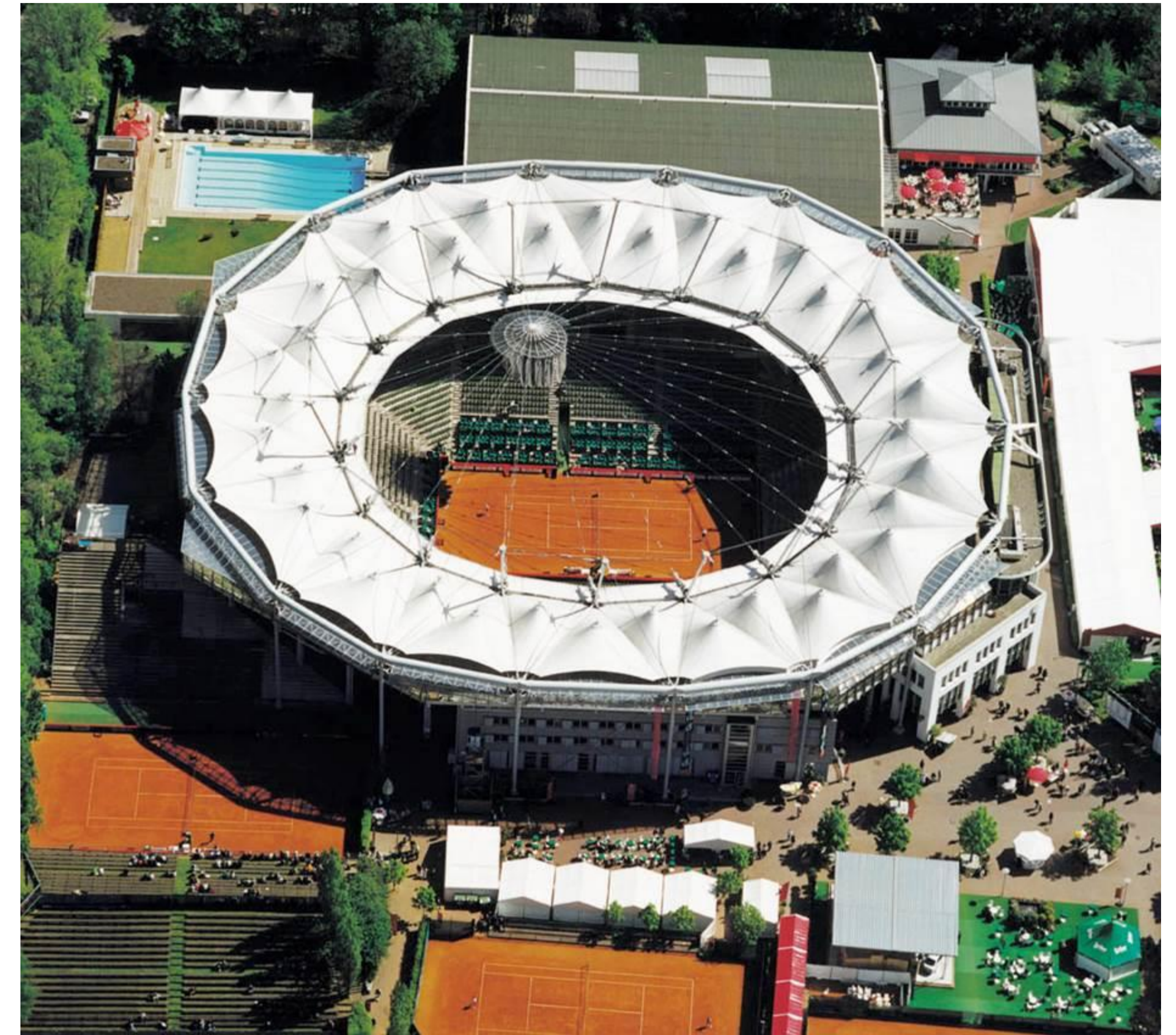
Figure 280) Exterior View, Open roof
