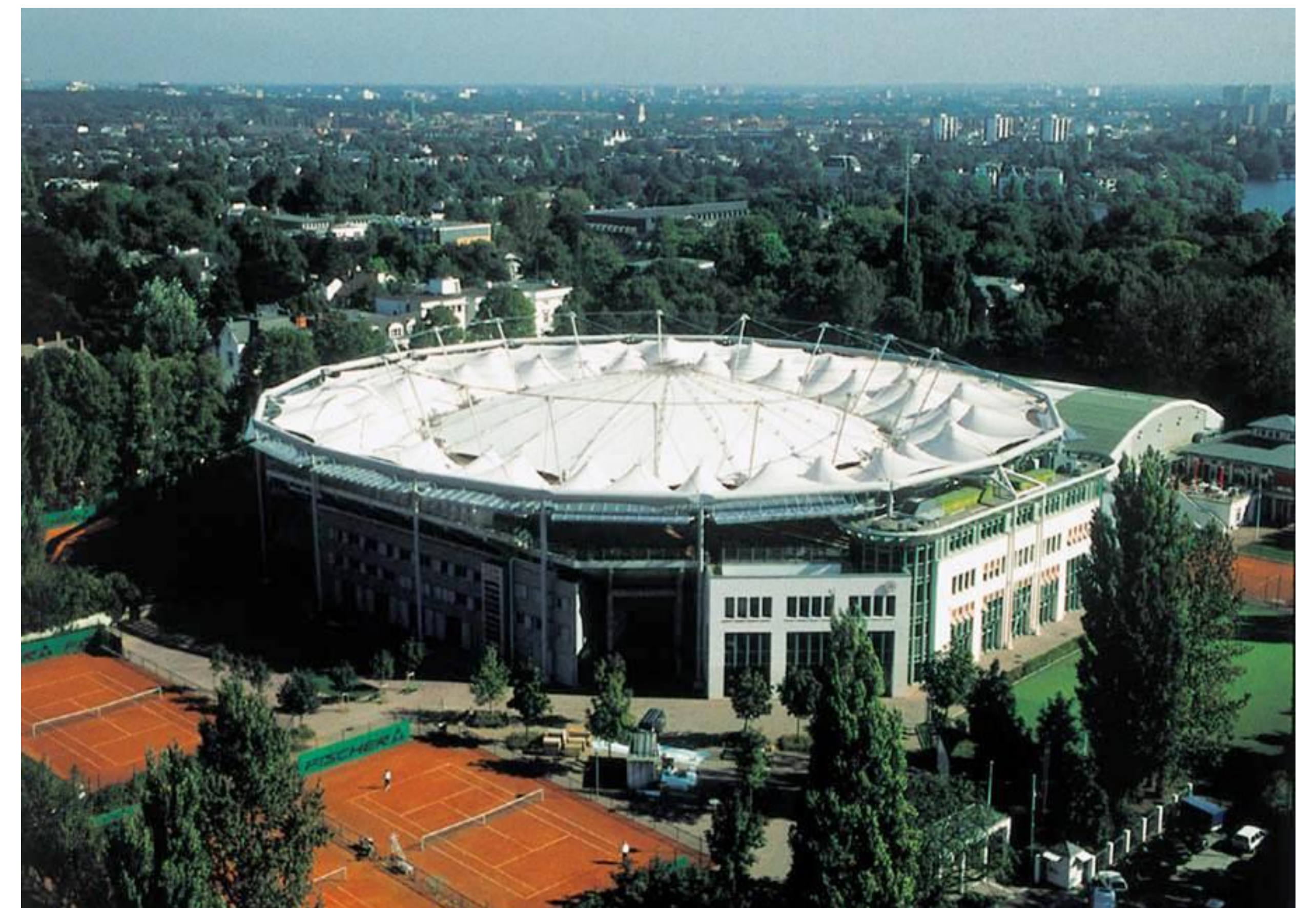
Figure 284) Exterior View, Closed roof
