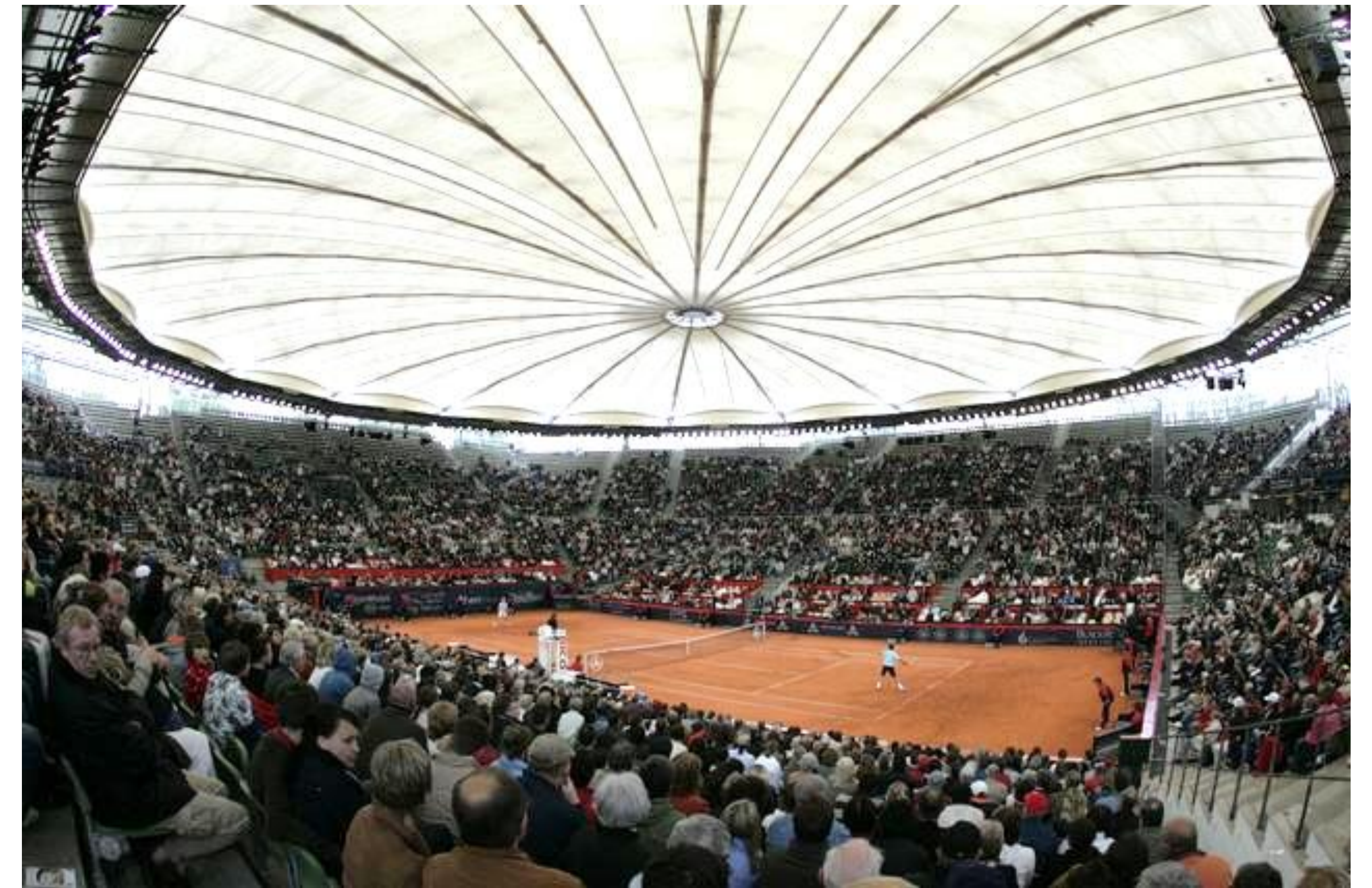
Figure 283) Interior View, Closed roof
