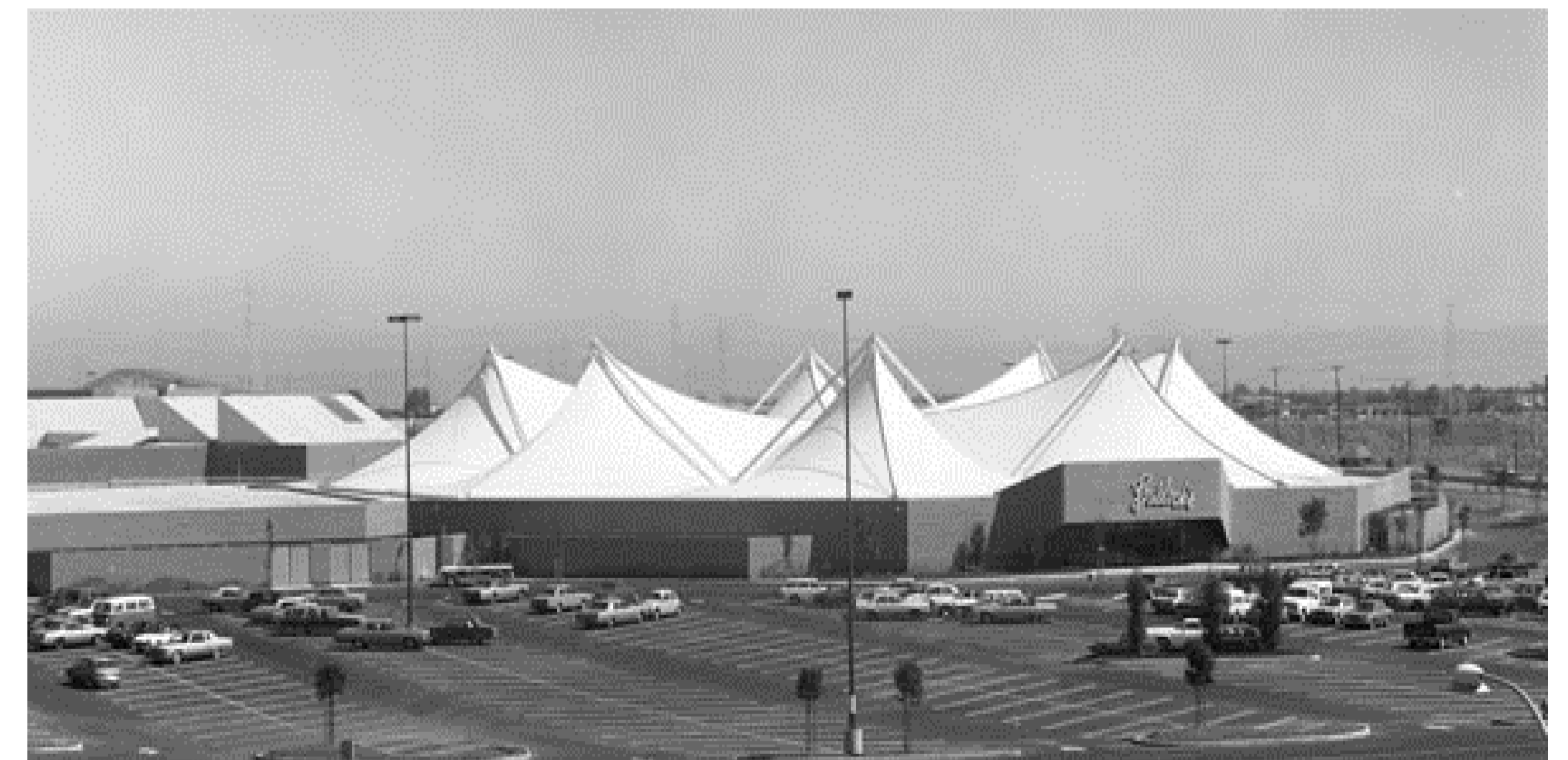
Figure 28) Florida Mall, an example of an American Large-scale tensile roof structure out of town
