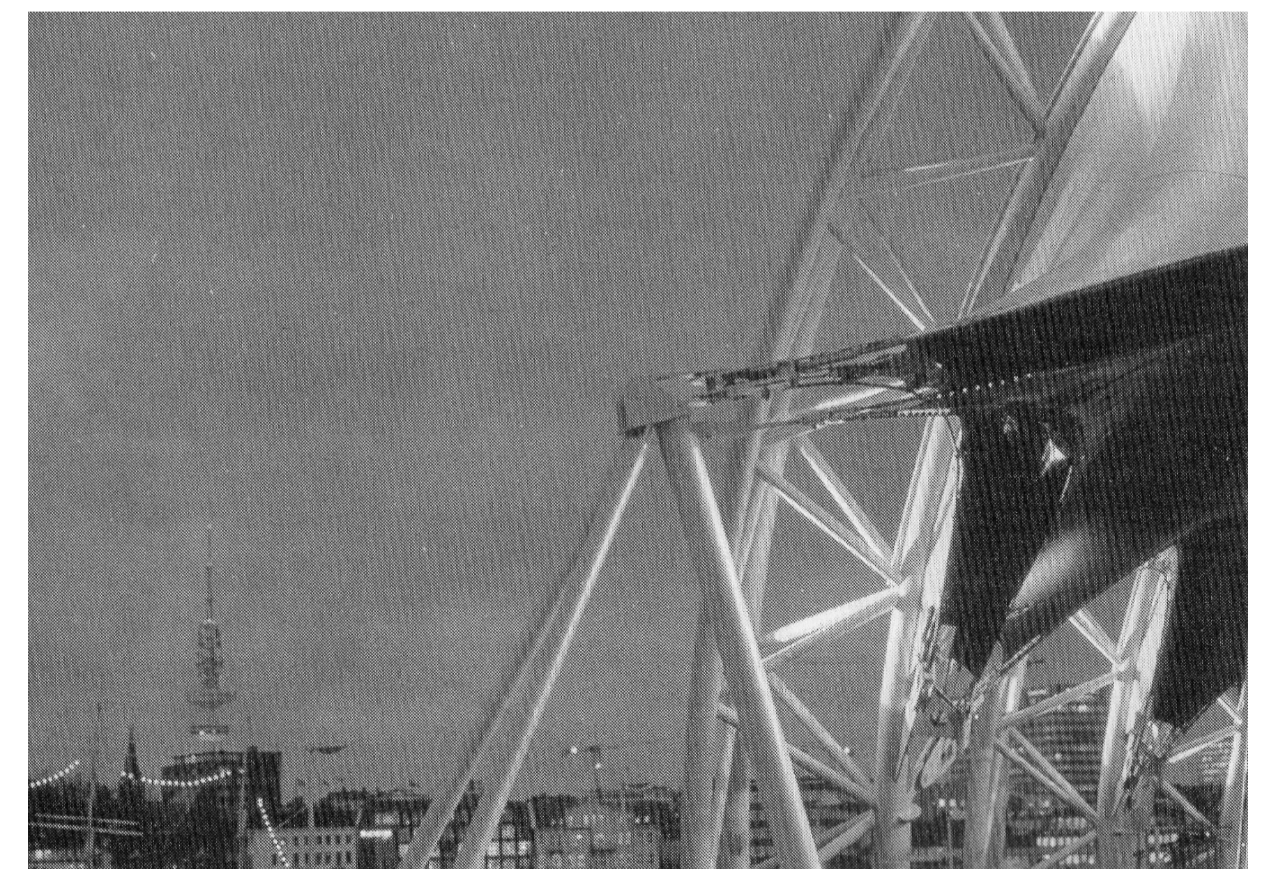
Figure 279) Membrane connection at tripod
