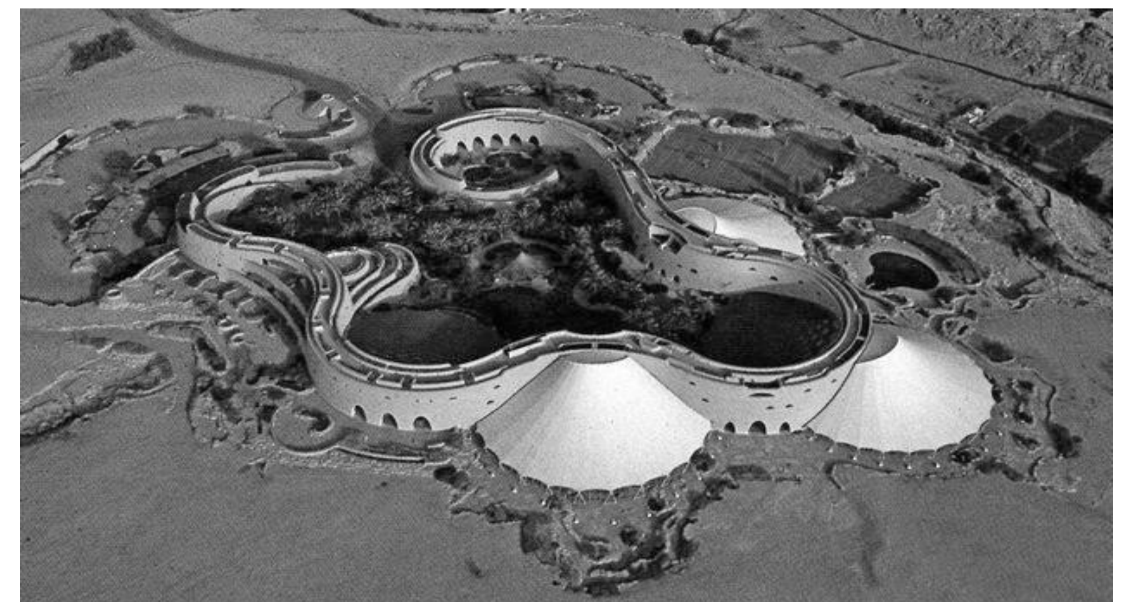
Figure 25) The Diplomatic club - Masonry Construction in combination with membrane structure and cable-nets, Riyadh 1986, Frei Otto
