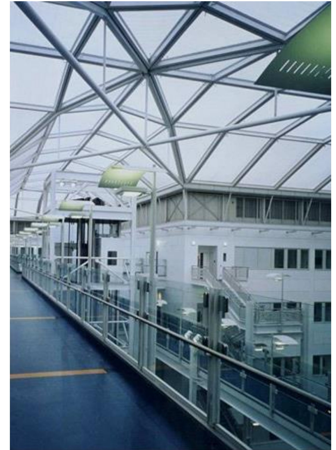
Figure 114) Interior View, The ETFE roof system allows maximum light transmission while retaining high insulation. Effective use of the Stack Effect enables easy ventilation of the central atrium space.
