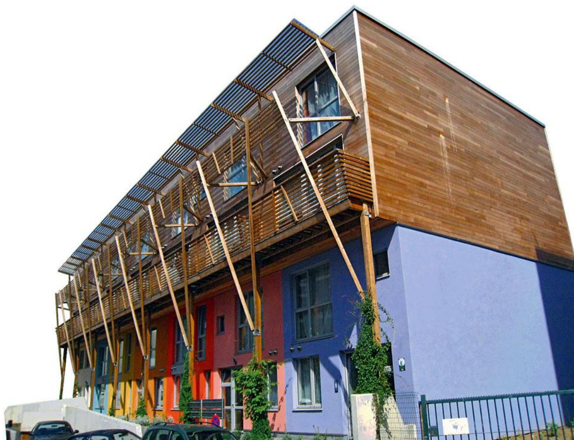
Fig.5.18. STREET VIEW OF THE PROJECT Source-Creating Cohousing: building sustainable communities / Kathryn McCamant and Charles Durrett
