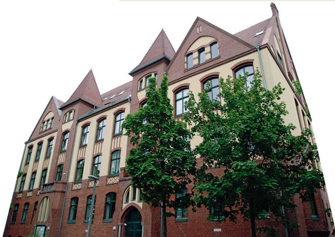
Fig.5.13. STREET VIEW OF THE PROJECT Source-Creating Cohousing: building sustainable communities / Kathryn McCamant and Charles Durrett
