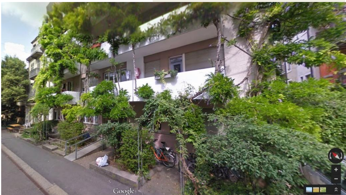
Fig.5.8. STREET VIEW OF THE PROJECT Source-www.designsponge.com
