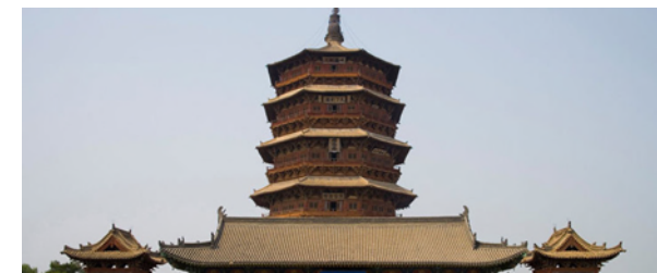
Fig.40 Wooden Tower of Ying County
