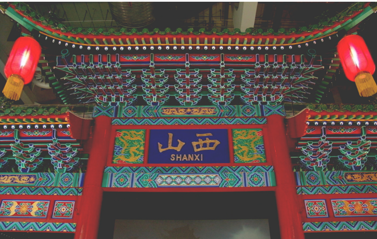
Fig.61 The Gate of Shanxi Pavilion
