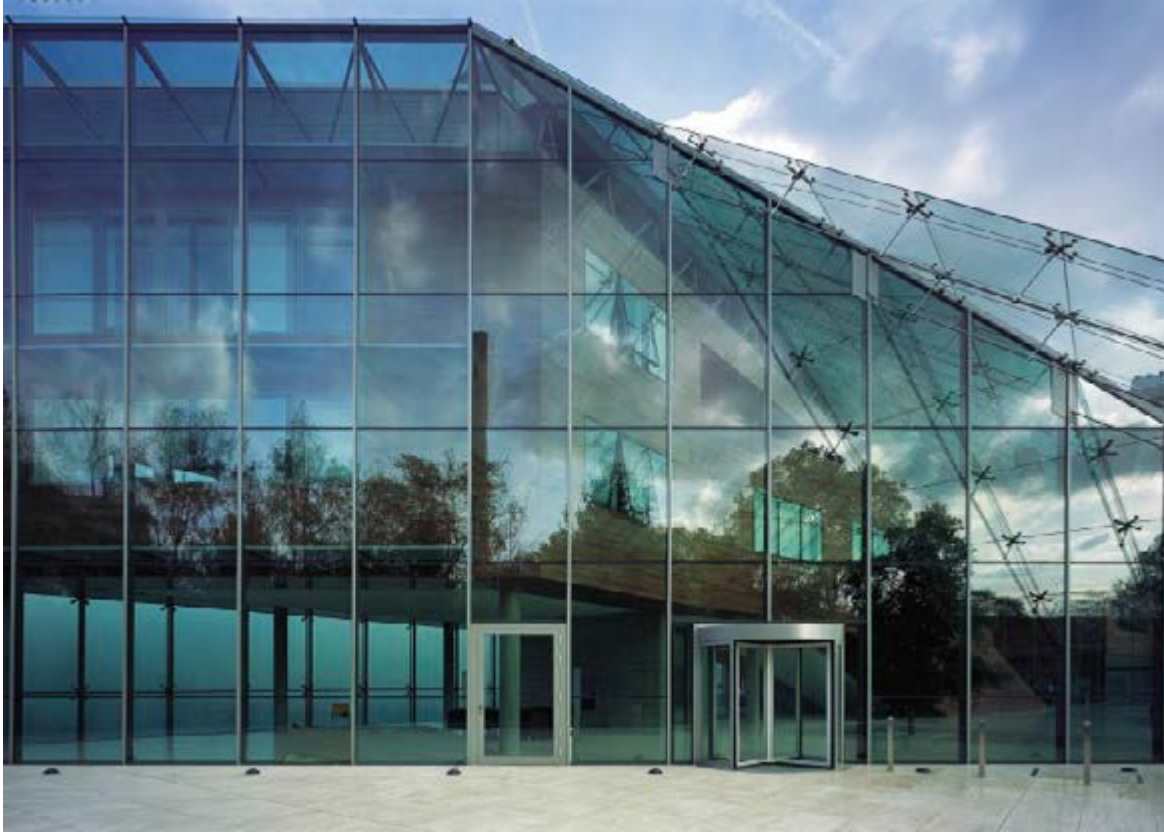
Hadi Mirmiran, General Consulate of Iran in Frankfurt, Frankfurt, 2004 View from the side of the building showing the rough volume suspended within a glazed case.
