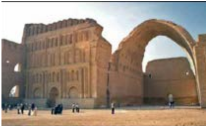
The Taq Kasra, meaning Iwan of Khosrau, is a Sassanid-era Persian monument in Al-Mada'in which is the only visible remaining structure of the ancient city of Ctesiphon. It is the largest brick built arch in the world and located near the modern town of Salman Pak, Iraq. Construction began DURING the reign of Khosrau I in 540 AD. The arched iwan hall, open on the facade side, was about 37 meters high 26 meters across and 50 meters long.
