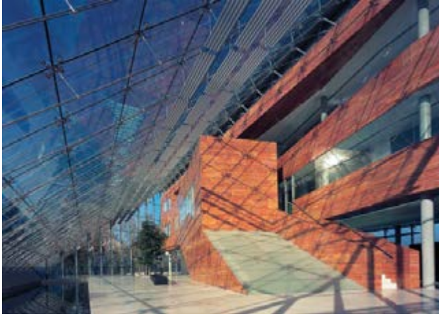
View of the multifunctional hall and glazed roof. The tree and line of water – elements borrowed from traditional Iranian architecture – create this transitional space between inside and outside.
