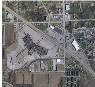
Fig. 141a,b-Immagine satellitare e schema di Southtown Mall, Fort Wayne, IN prima del demalling Fig. 141a,b-Satellite image and scheme of Southtown Mall, Fort Wayne, IN before the demalling
