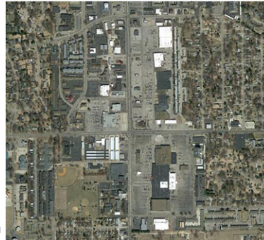
Fig. 140a,b-Immagine satellitare e schema di Washington Square Mall, Evansville, IN prima del demalling Fig. 140a,b-Satellite image and scheme of Washington Square Mall, Evansville, IN before the demalling
