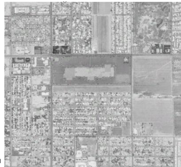
Fig. 113a,b-Immagine satellitare e schema di Valley West Mall, Glendale, AZ prima del demalling Fig. 113a,b-Satellite image and scheme of Valley West Mall, Glendale, AZ before the demalling
