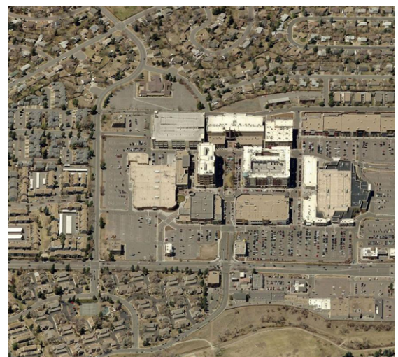
Fig. 018-Town center mixed use con The Streets at SouthGlenn in Centennial, CO Fig. 018-Town center mixed use with The Streets at SouthGlenn in Centennial, CO
