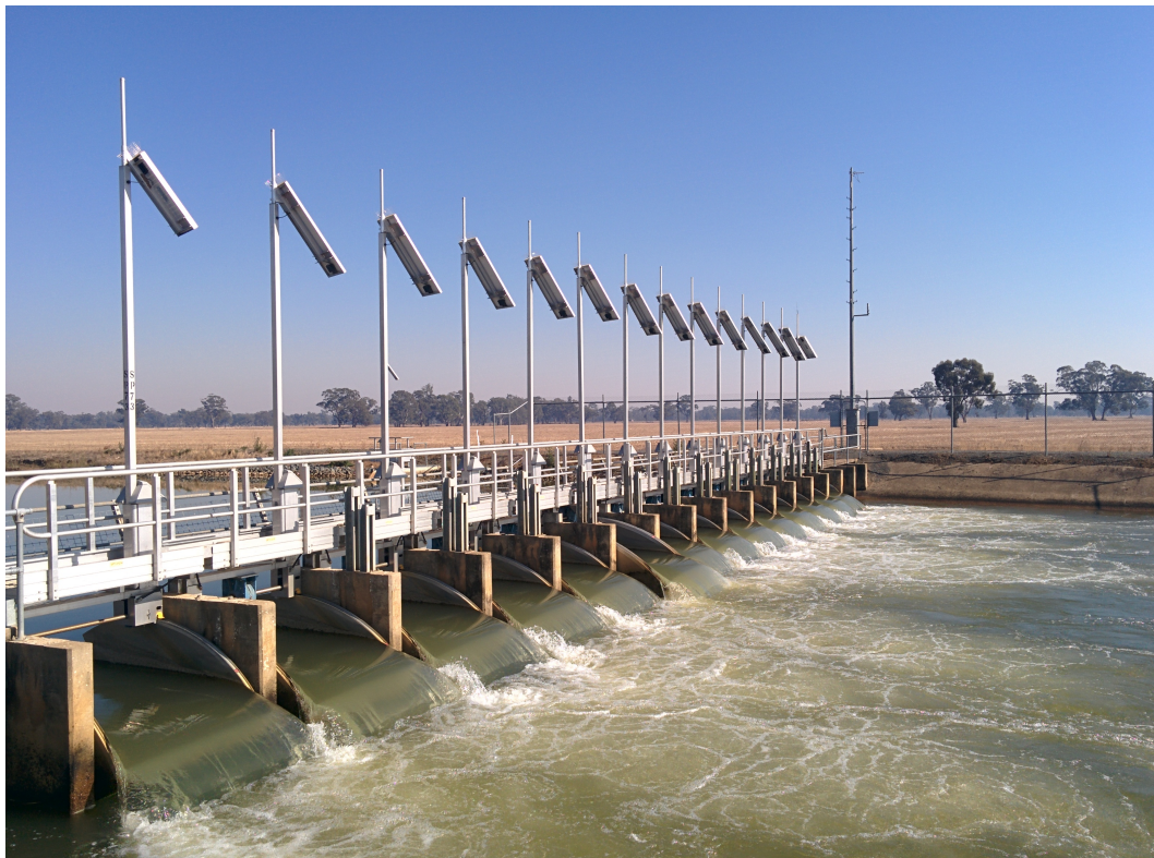
Figure 1.1: Irrigation Channel: focus on a gate
