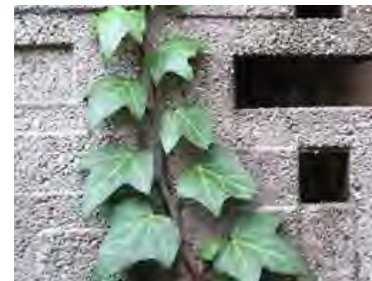
Millard House wall detail, Frank Lloyd Wright
