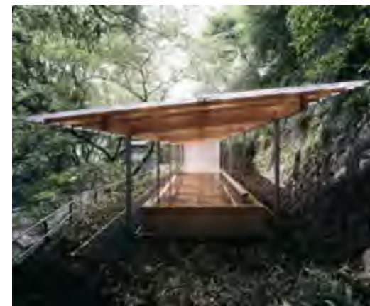
Horai Onsen Bathhouse, Kengo Kuma
