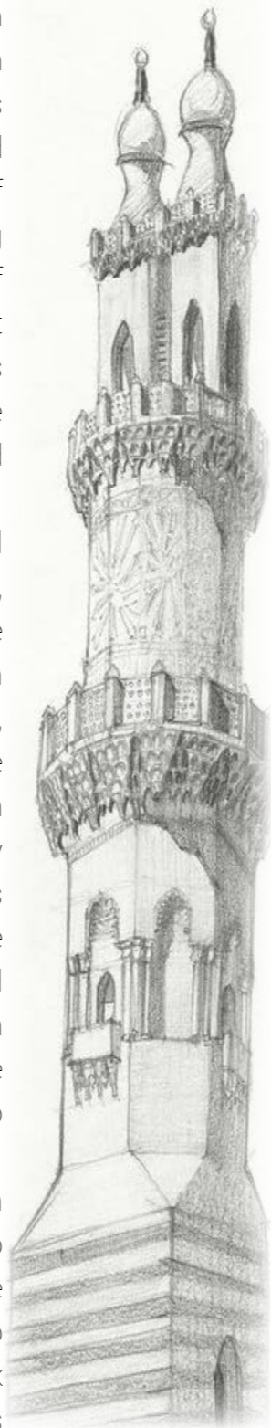
Fig. 61: Minaret of Al-Azhar mosque added by Sultan Al-Ghuri. 61
