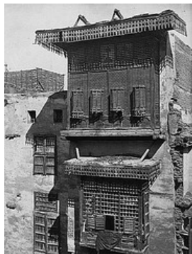
Fig. 28: Picture showing the Mashrabiyya on the facade of one of the Cairene houses.
