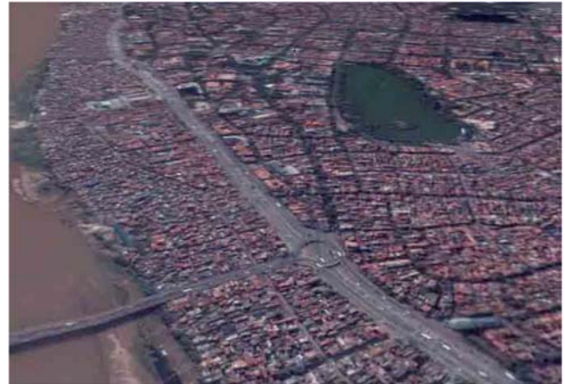
Present: The riverside is encroached by illegal houses
