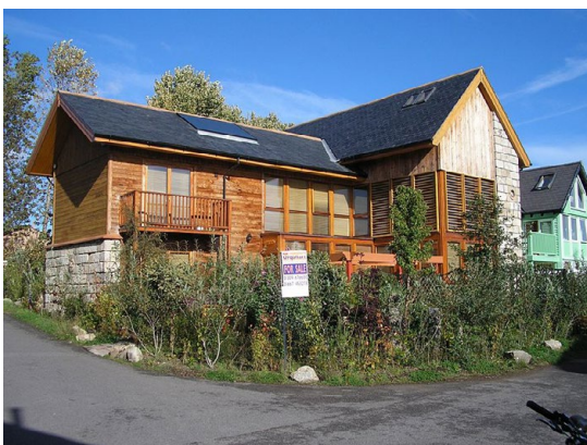
Figure 3.6 : A 200 m 2 plus Eco-house in Findhorn Ecovillage, Scotland. [1]
