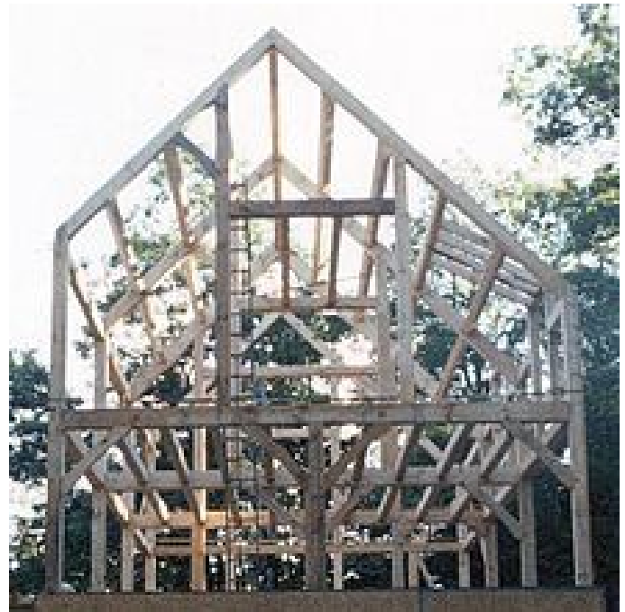
Figure 2.31 : The completed frame of a modern timber frame home. [63]
