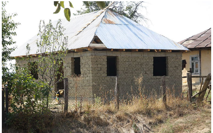
Figure 2.20 : Adobe brick house under construction in Romania. [50]
