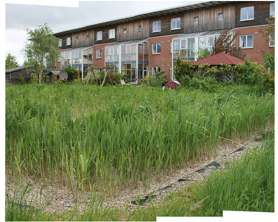
Figure 2.43 : Constructed wetland in an ecological settlement in Flintbreite near Luebeck, Germany. [79]
