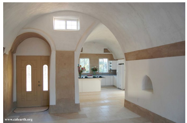
Figure 2.25 : A house built with earthbag construction. Image source: www.calearth.org
