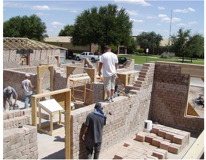
Figure 2.22 : Building a CEB project in Midland, Texas in August 2006 [53]
