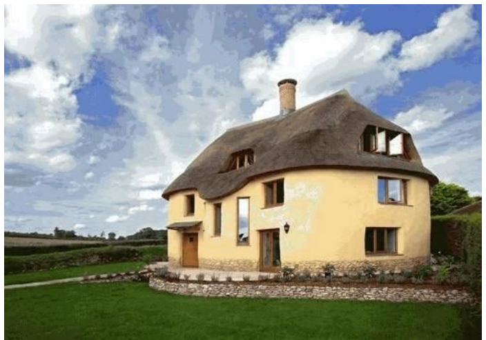
Figure 2.21 : A modern cob house near Ottery St Mary in the United Kingdom. [51]
