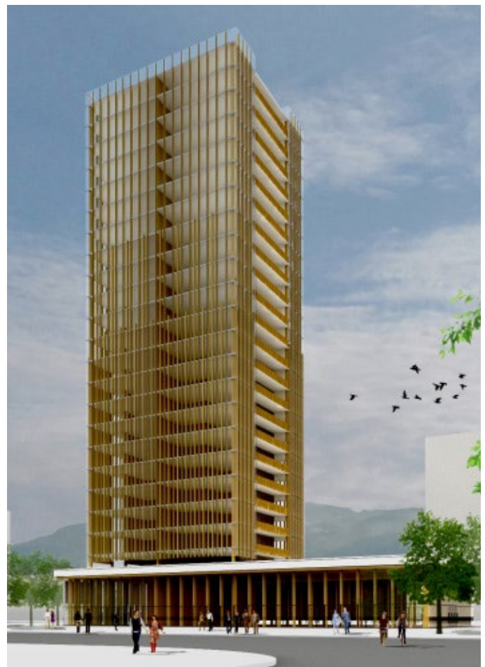
Figure 2.32 : Michael Green's hypothesis for a 30 storey skyscraper with a mass timber panels structural frame and a glulam curtain wall. [64]
