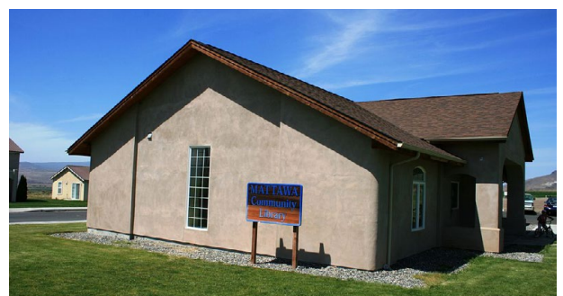
Figure 2.29 : Exterior view of straw bale library in Mattawa, Washington taken in 2008 (constructed 2002 by IronStraw Group) [59]
