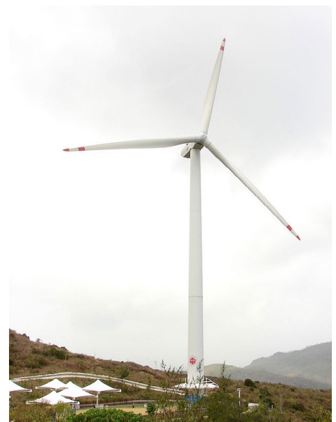
Figure 2.39 : The Nordex N50 wind turbine and visitor centre of Lamma Winds in Hong Kong, China. [71]
