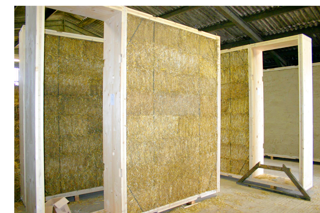
A photo of a prefabricated ModCell® panel wall system in assembly
