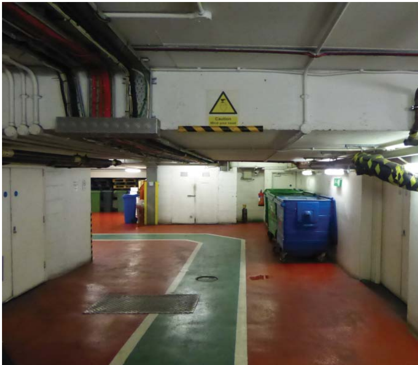
Fig. 168 "(top) Ceiling height is extremely restricted in thebasement. This area is shown at 2.4 m. To the right of the columns the ceiling height is 2m. (Bottom left) The existing structure creates a low ceiling height of 2m is indicated in the photo, taken at the bottom of the ramp. (Bottom right) Market expectations of cycling changing facilities."
