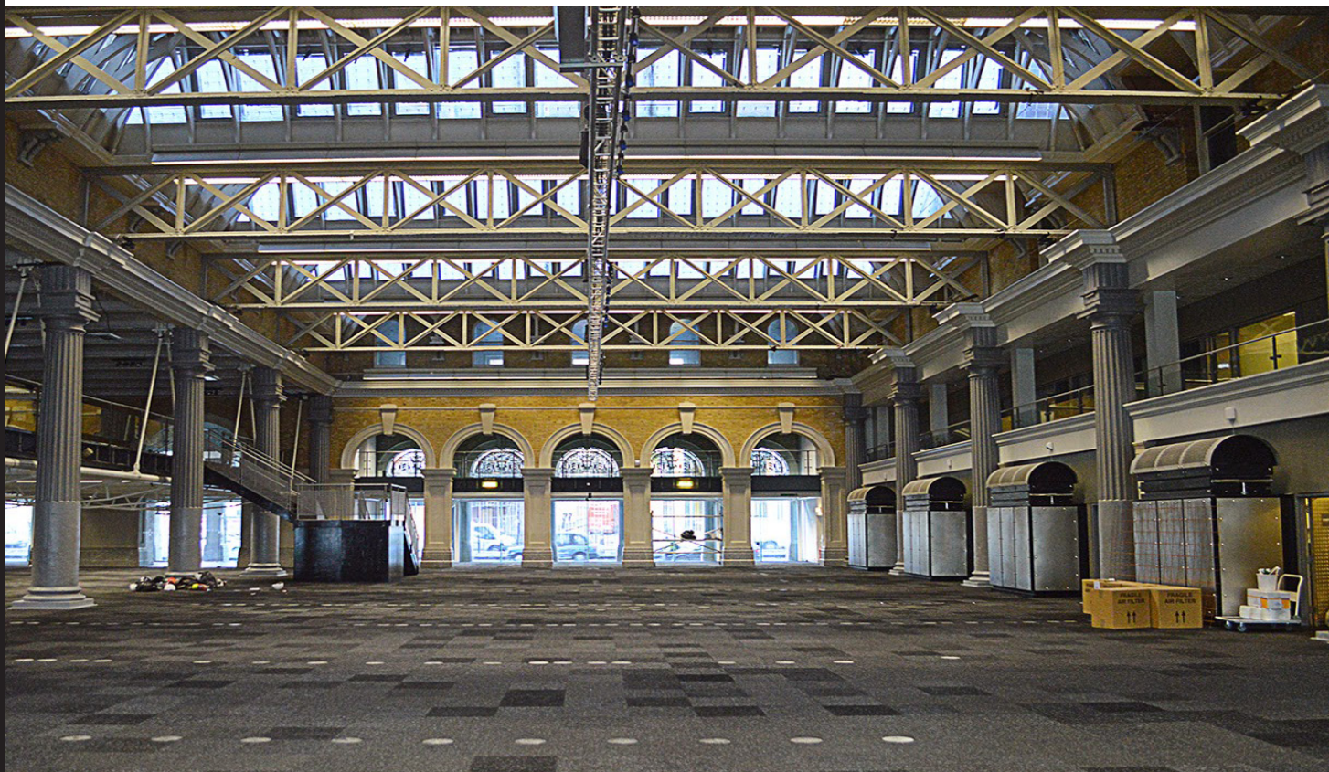
Fig. 91 "Main hall of the building" Source: www.rsh-p.com
