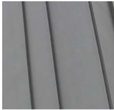
Dark grey zinc roofing
