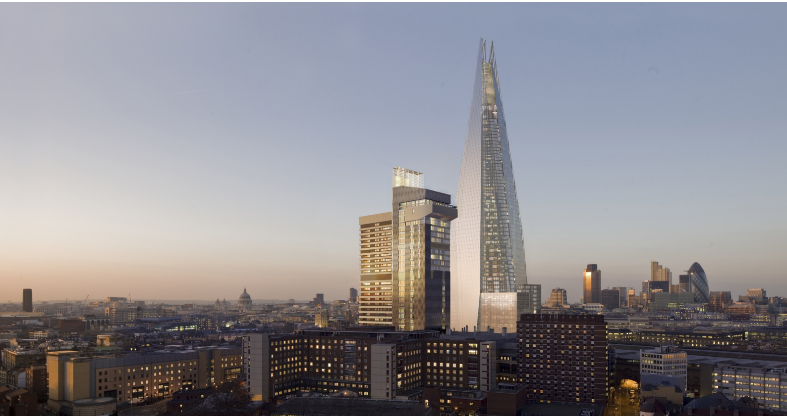
Fig.106 "View of Guy's Tower after the refurbishment with the Shard at the back" Source: Peynore&Prasad website
