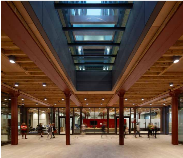
Fig. 66 "The Granary: ground floor. Red-wrought iron columns, raw timber, and a new glazed stairwell punched through the building" S: S. Williams
