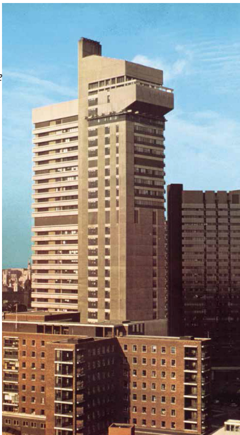
"Link bridge between the two towers"
