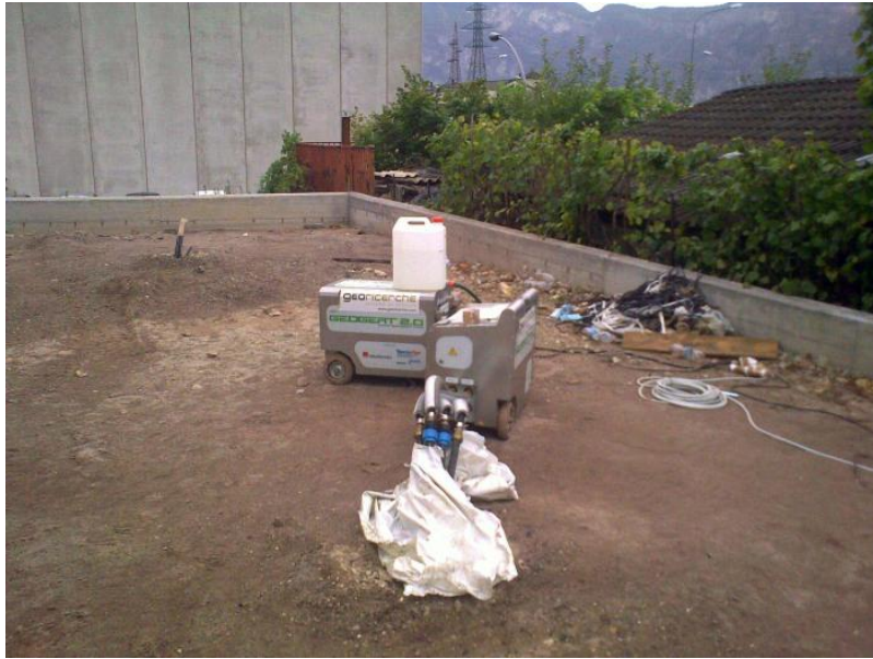
Figure 4-4 - Connection of the two delivery pipes and two runback, GEOgert 2.0.
