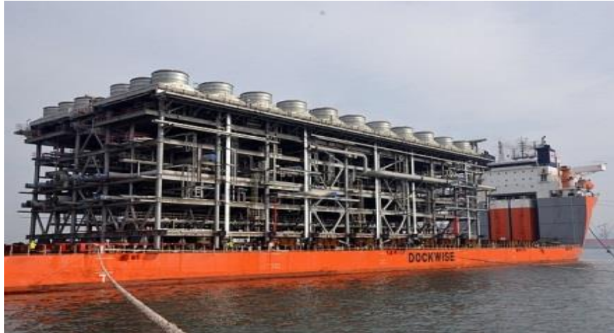
Figure 3 - Figure 4 - Pipe rack module
