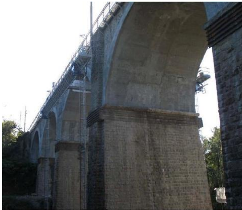
Figure 2.6 – Bridge structure with scaffolding (Nanni 2013)
