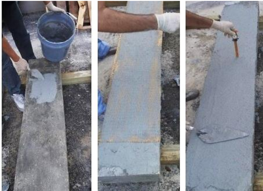
Figure 2.5 – Demonstration of installation procedure of FRCM strengthening
