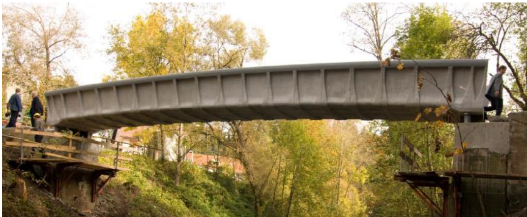
Figure 1.3 – 17 meter bridge made of TRC in Kempten (Allgäu)
