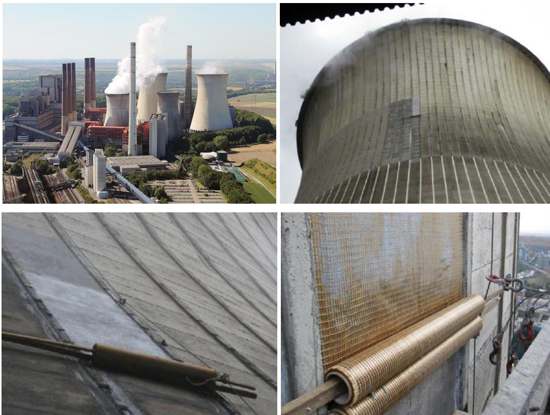
Figure 2.11 – Strengthening of cooling towers (Germany)
