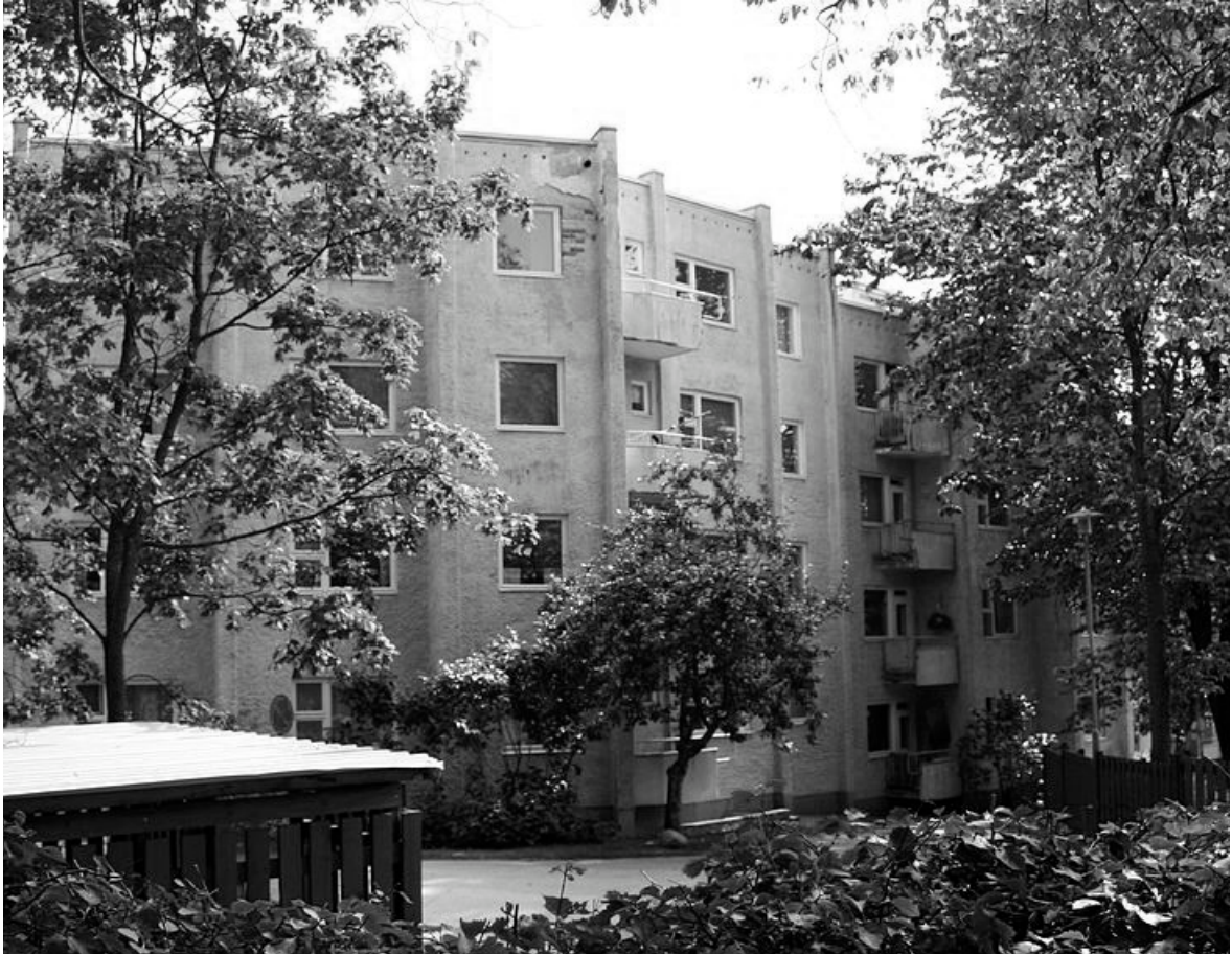
"Serpentine House" housing block, Helsinki, Yrjö Lindegren, 1949-51.
