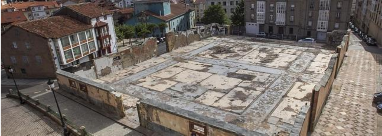
Figure 2.28 Site after fire
