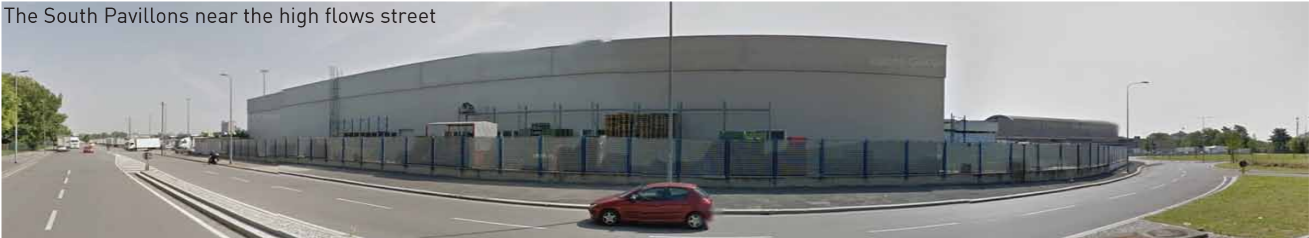
Another 'gated' view about existing logistic pavillons
