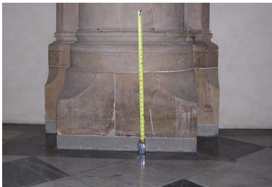
Figure 8 Base Group 3 Pier (5 West)
