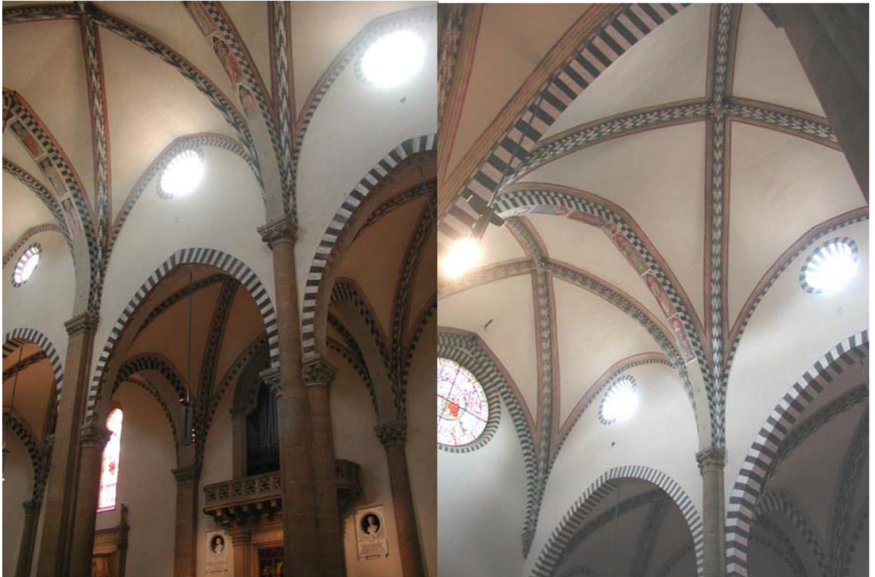
Figure 6 Vault ribs over 4-lobed pier
