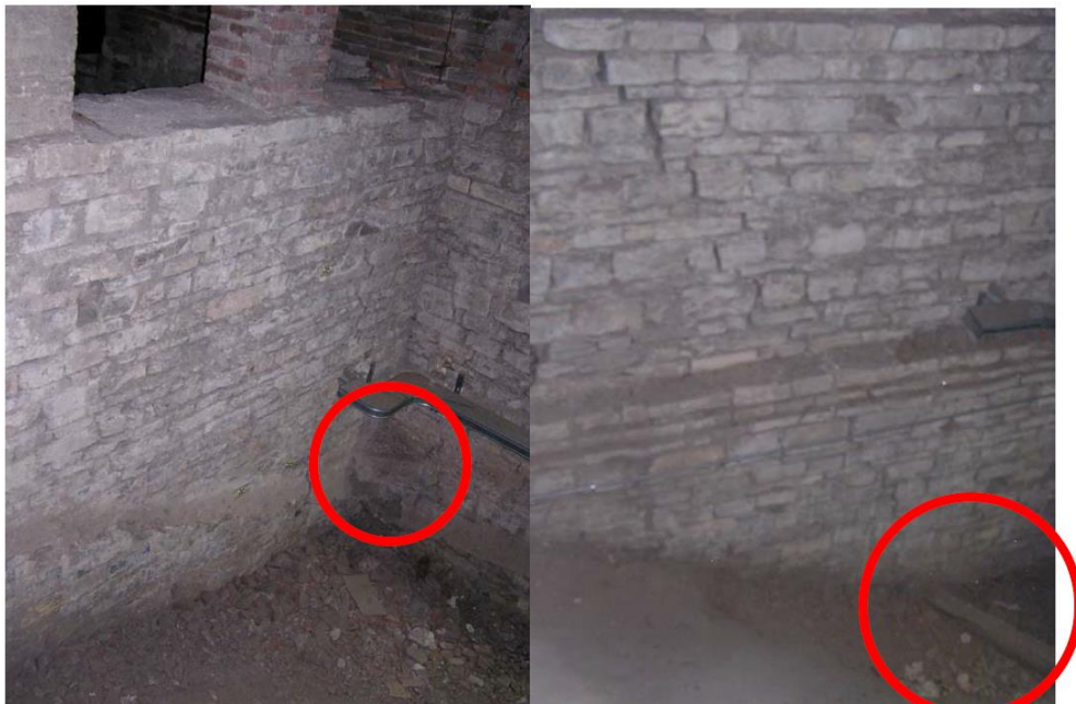
Figure 13 Wall between nave bays 4 and 5
