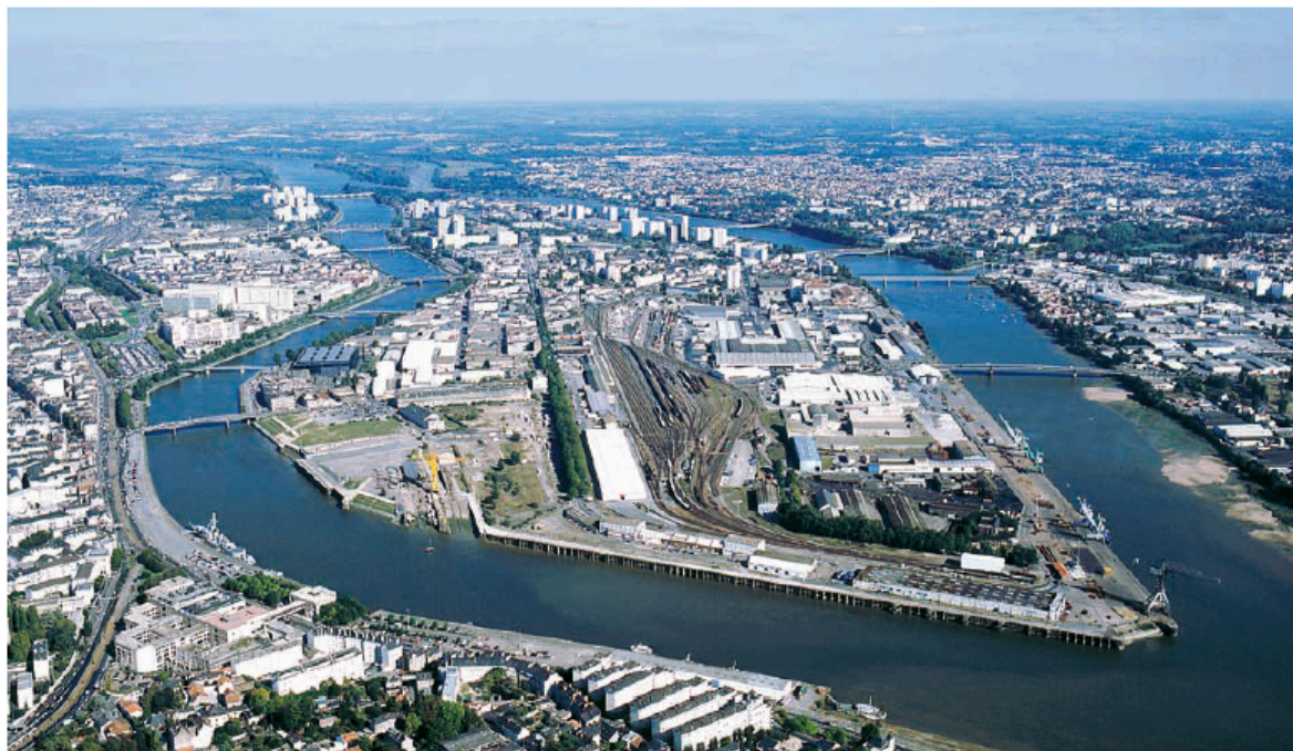
Figure 4: Aerial view of the Ile de Nantes and the railway site of Nantes Etat right in the middle
