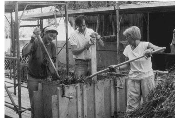
MAKING LIGHTWEIGHT STRAW LOAM BLOCKS
