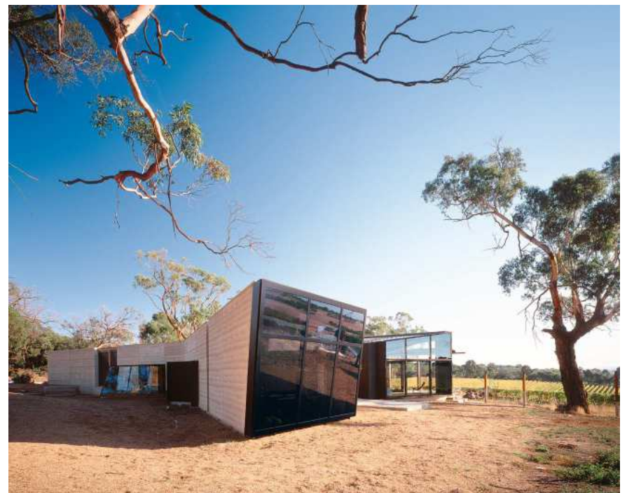
VINEYARD RESIDENCE AT MORNINGTON PENINSULA, VICTORIA, AUSTRALIA
