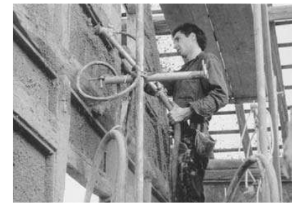
SPRAYING LIGHTWEIGHT LOAM
