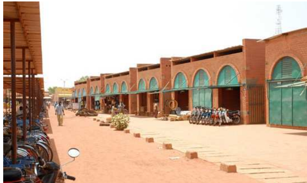
SHUTTERS THAT CLOSE THE STALLS AT NIGHT ACT AS SHADINGS DURING THE DAY
