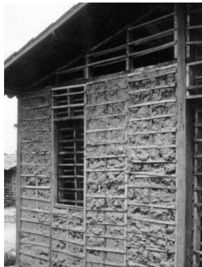
PREFABRICATED WATTLE-AND-DAUB SYSTEM, BRAZIL
