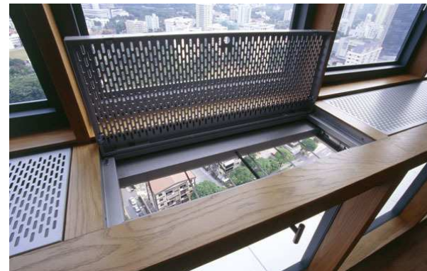
THE TRADITIONAL MONSOON WINDOW AT THE MOULMEIN RISE RESIDENTIAL TOWER IN SINGAPORE
