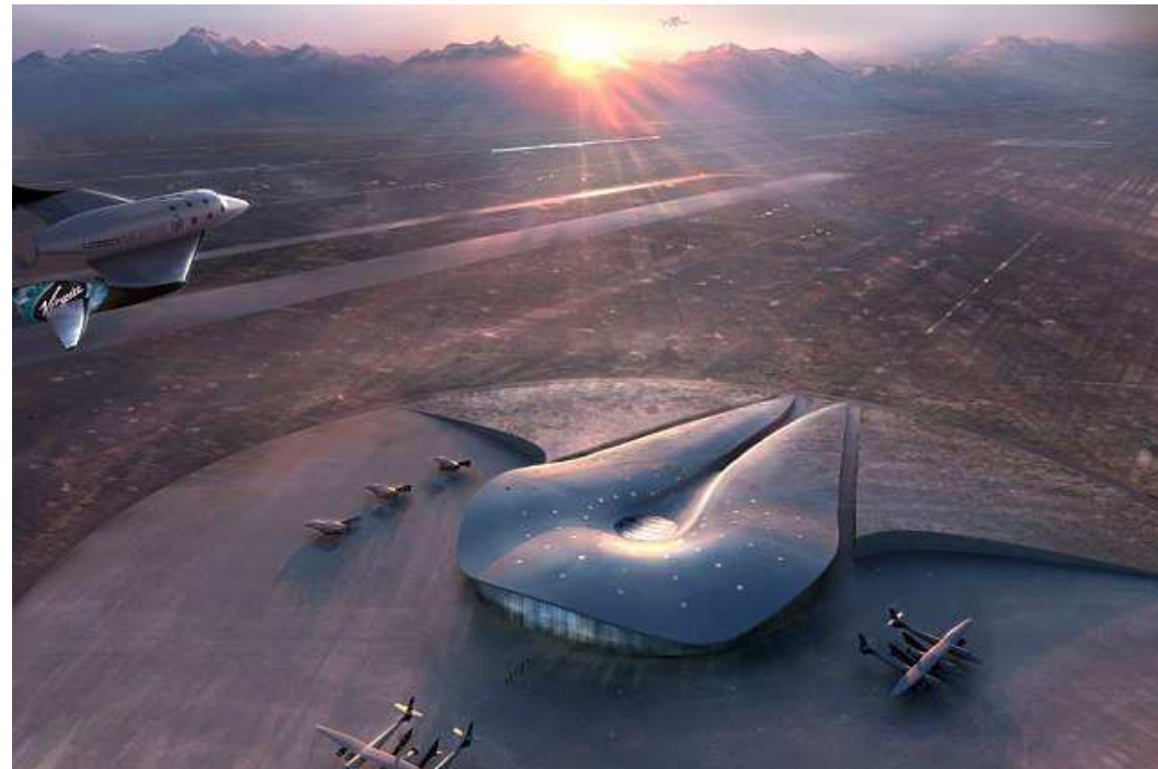
VIRGIN GALACTIC'S SPACEPORT AMERICA UNDER CONSTRUCTION IN THE DESERT OF NEW MEXICO DESIGNED BY NORMAN FOSTER
