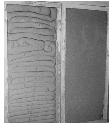
STRUCTURAL ELEMENTS FILLED WITH LIGHT WEIGHT LOAM
