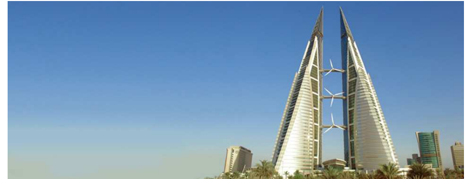
WIND TURBINES ON ATKINS' WORLD TRADE CENTRE IN BAHRAIN GENERATE BETWEEN 10-15% OF THE TOTAL ENERGY REQUIREMENT
