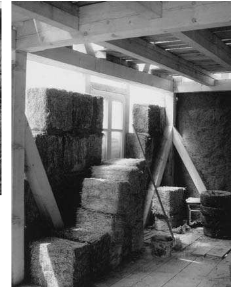
EXTERIOR WALL MADE OF LARGE BLOCKS OF LIGHTWEIGHT STRAW LOAM
