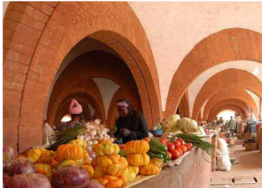
THE MARKET'S VAULTED DOMES FORM A RECTANGULAR GRID
