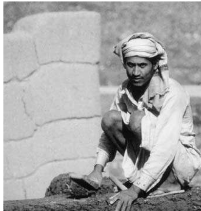
CONSTRUCTION OF A LOAM WALL, USING THE ZABUR TECHNIQUE, YEMEN
