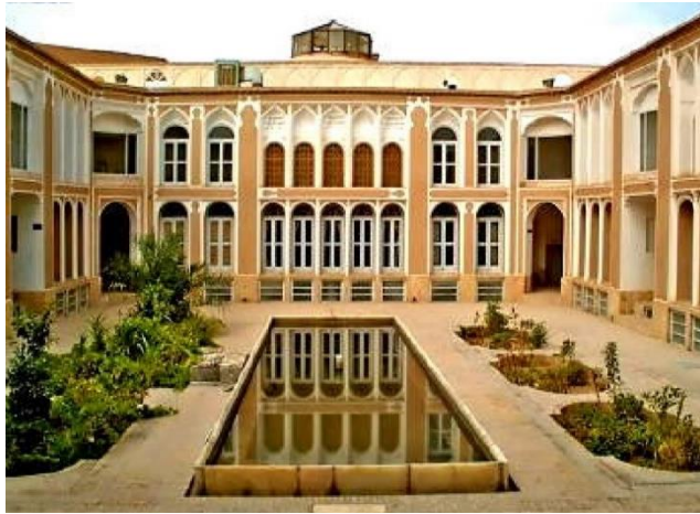
Fig.6.3. Court Yard of Mortas House, in Yazd, shows connection of the human and nature
