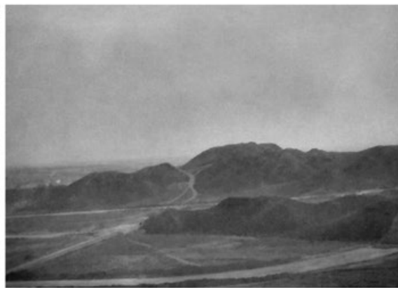
Figure 11, Placing part of the project between the existing hills
