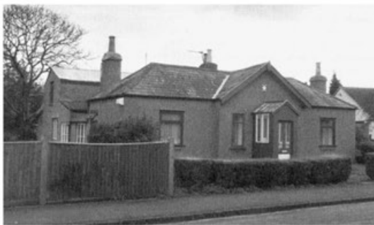
Figure 03, Cottage cum smallholding at Minster Lovell in Oxford shire, one of several settlements built by the Chartist Land Company to provide working people with an escape route from the industrial city
