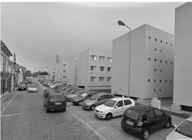
Figure 43, Rua daSeara Matosinhos, PER, 1999-2000 João Álvaro Rocha
