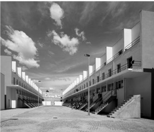
Figure 68, View to the public space
