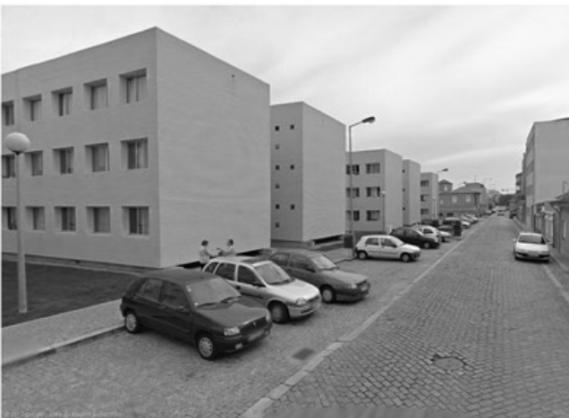
Figure 42, Rua daSeara Matosinhos,PER, 1999-2000, João Álvaro Rocha
