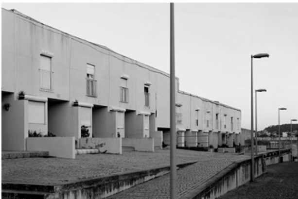
Figure 64, View to the public space
