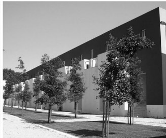
Figure 69, View to the public space
