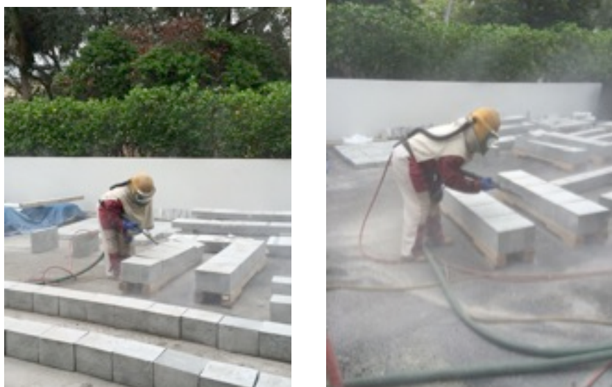
Fig. 2. 16 - Sandblasting performed by a professional operator
