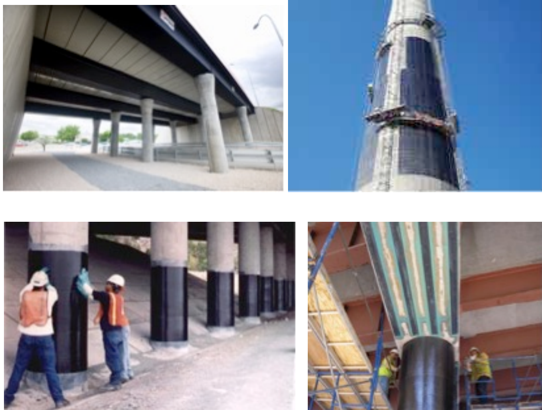
Fig. 1. 4 - Some Application of FRPs
