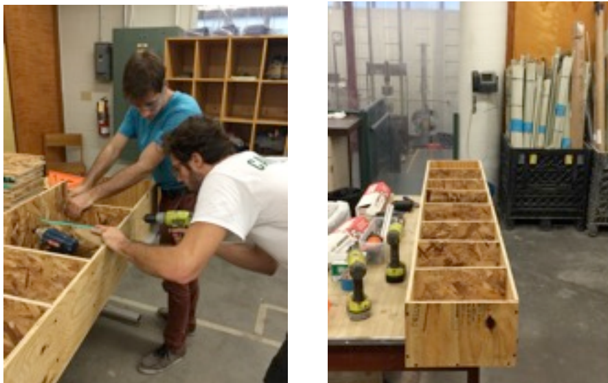
Fig. 2. 12 - Wooden mold construction
