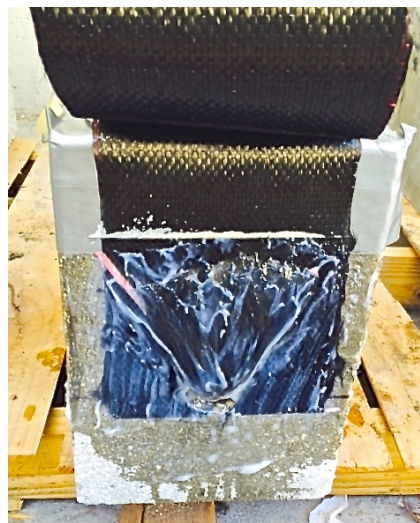
Fig. 2. 46 - Specimen after the application of the thickened epoxy
