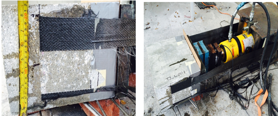
Fig. 3. 6 – Failure Mode A
