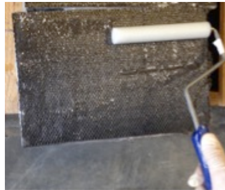
Fig. 2. 32 – Installation (left) and rolling (right) of the FRP sheet
