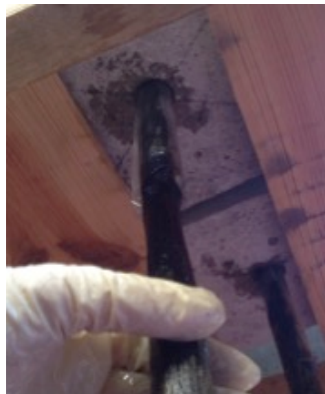
Fig. 2. 36 - Insertion of the anchor inside the tube
