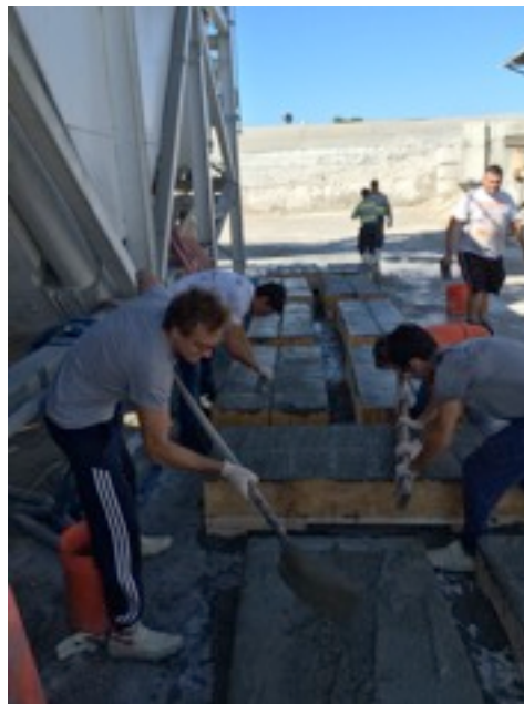
Fig. 2. 15 - Casting of the concrete
