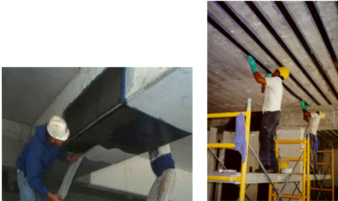
Fig. 1. 1 – Application of FRPs
