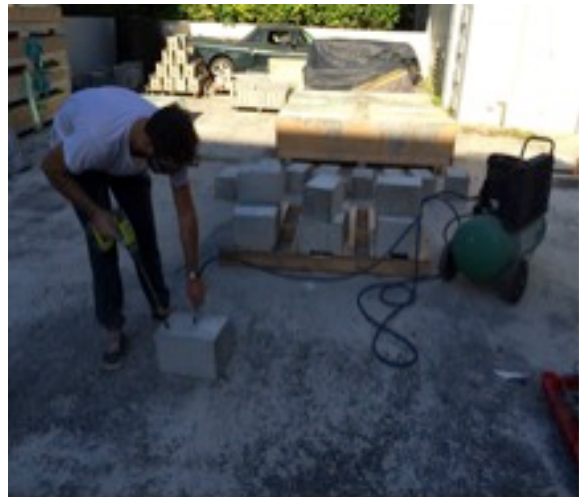
Fig. 2. 21 - Operation of cleaning the hole
