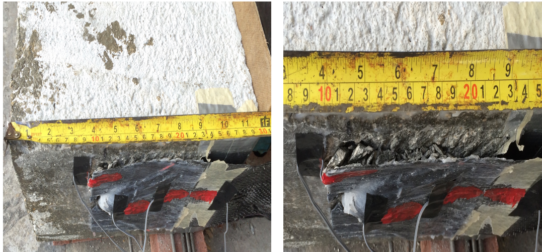
Fig. 3. 9 – Observed Failure Mode D
