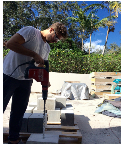
Fig. 1. 19 - Operation of drilling
