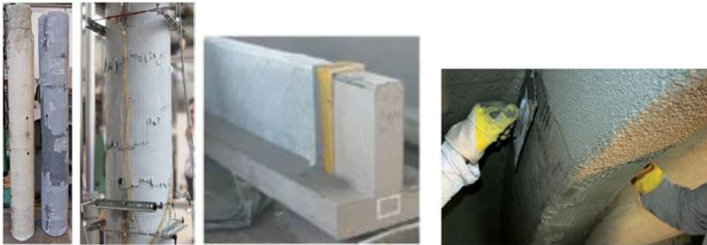
Figure 2.17: Applying TRC layers to different structural items [Curbach and Sheerer 2011].
