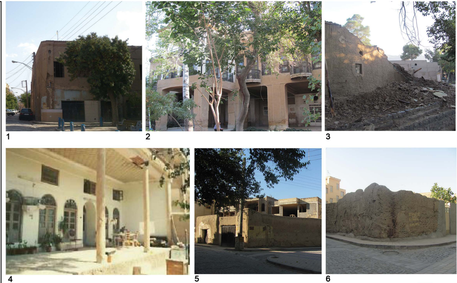
Figure 40; historical buildings to be reused or demolished Ref: Ministry of Culture and Art
