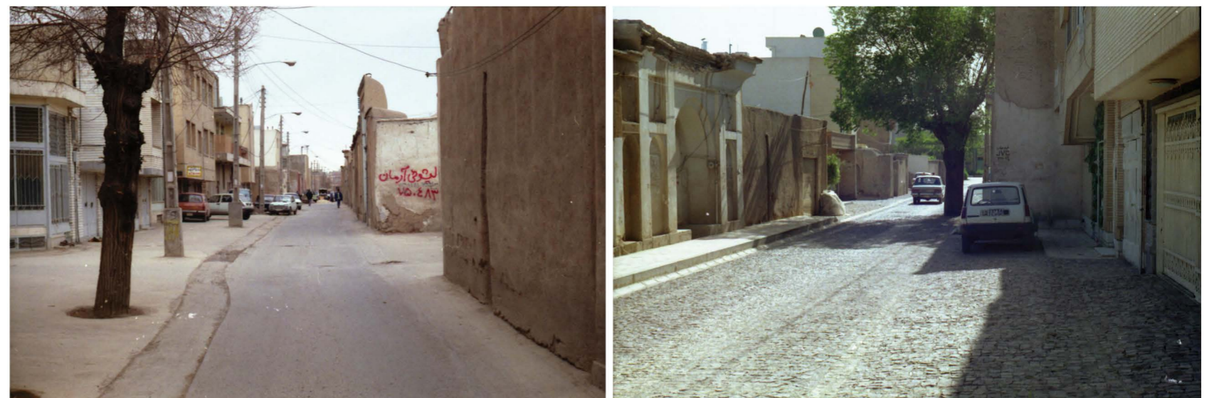
Figure 31; change of pavement in Sangtarashha Street; left: before restoration/ right: after restoration Ref: municipality of Isfahan
