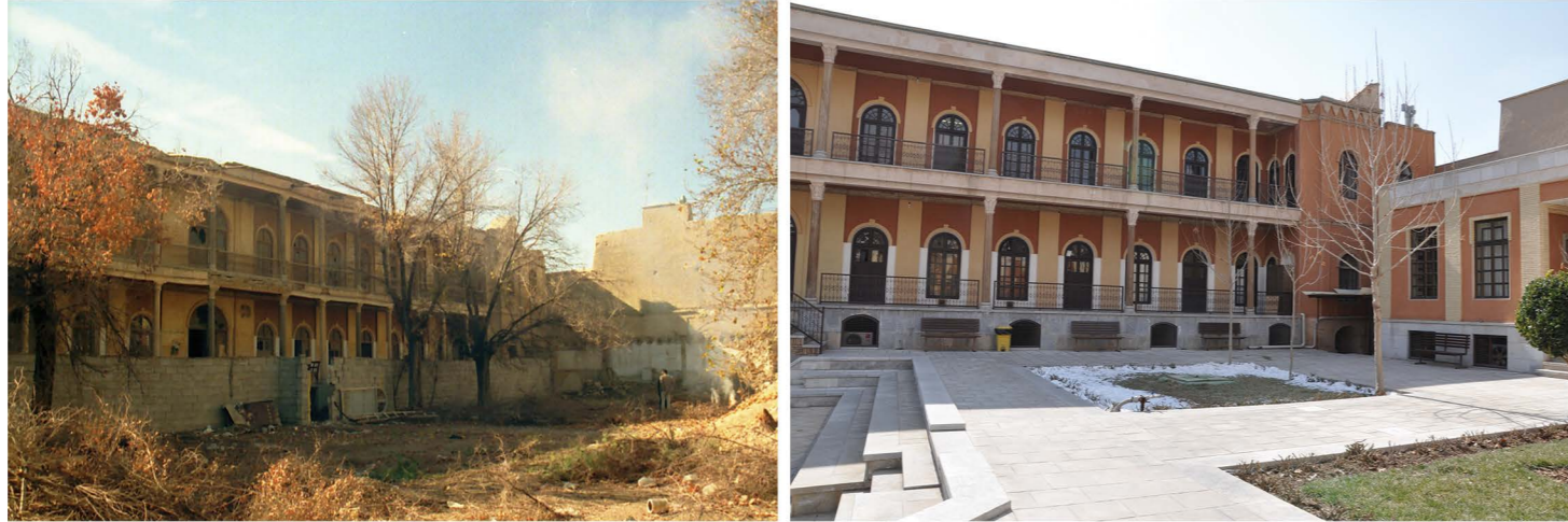
Faransaviha School; left: before restoration/ right: after restoration
