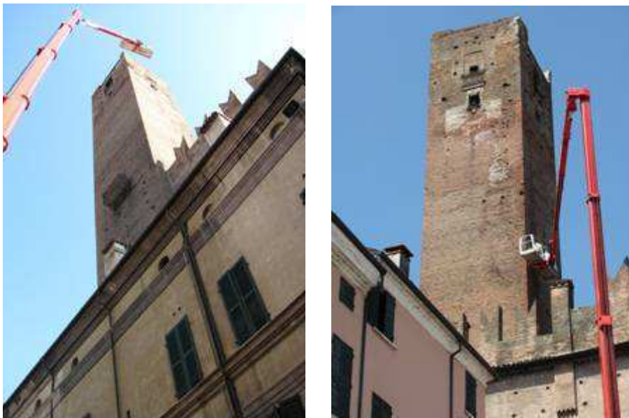
Figure 4.6 Visual inspection of the tower using a movable platform
